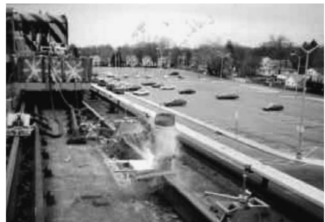
Figure 3. Test welds installation and welder training.
