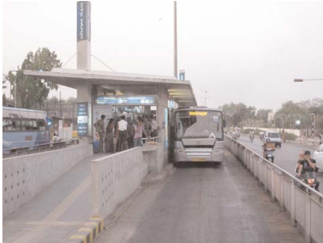
Figure 1 BRT station in Ahmedabad.
