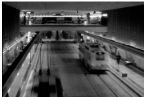
Seattle Bus Tunnel
