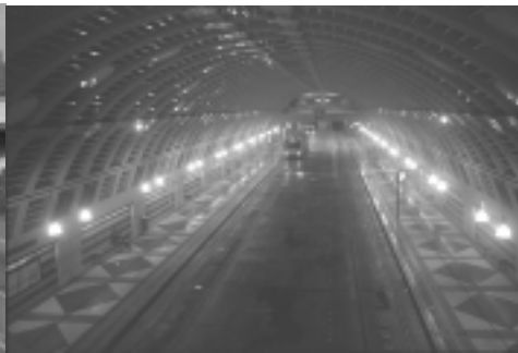
Seattle Bus Tunnel
