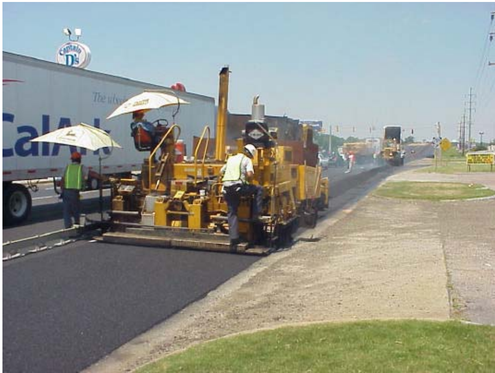
Figure 35 – Paver equipped with “shuttlebuggy” for PG 82-22 paving
