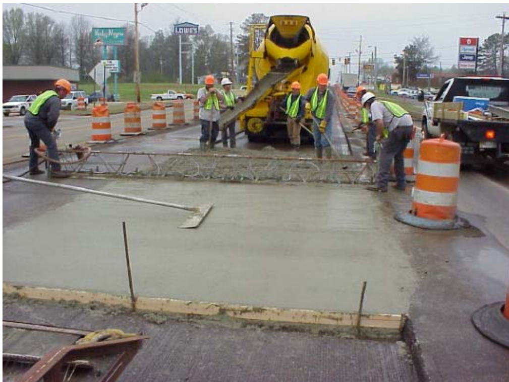
Figure 11 – Pouring concrete at the Ultra-Thin Whitetopping test section
