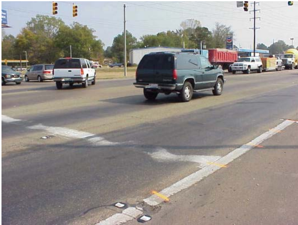
Figure 5 – Intersection of US 72 and Cass Street (looking east)
