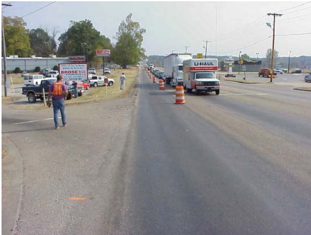
Figure 7 – Intersection of US 72 and Hinton Street (looking east)
