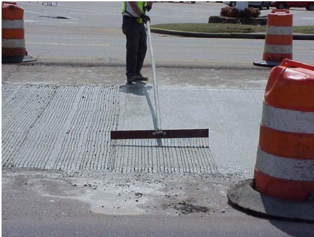
Figure 12 – Whitetopping is given a transverse tined finish with a metal broom
