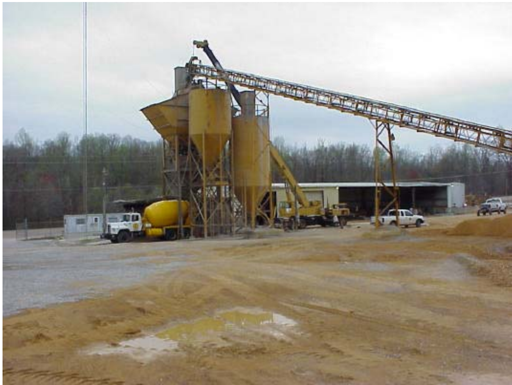
Figure 20 – B & B Concrete Corinth plant which supplied the grout for the RMP
