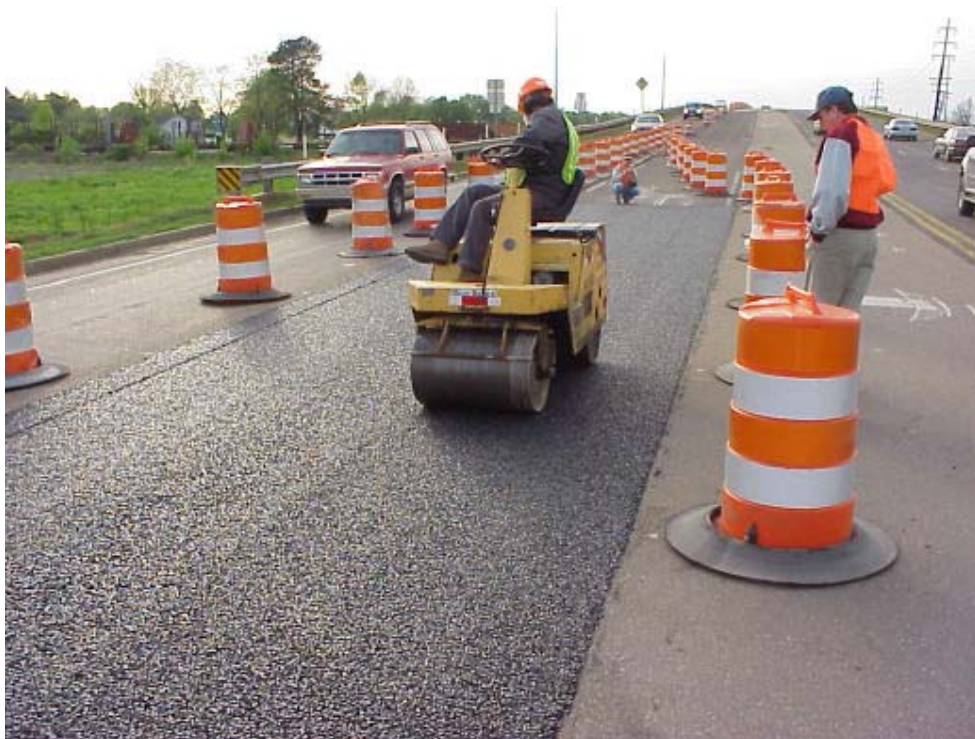
Figure 19 – Open graded mix is subjected to one pass with a 1½ ton roller in static mode @ approximately 150 degrees F to “seat” the aggregate
