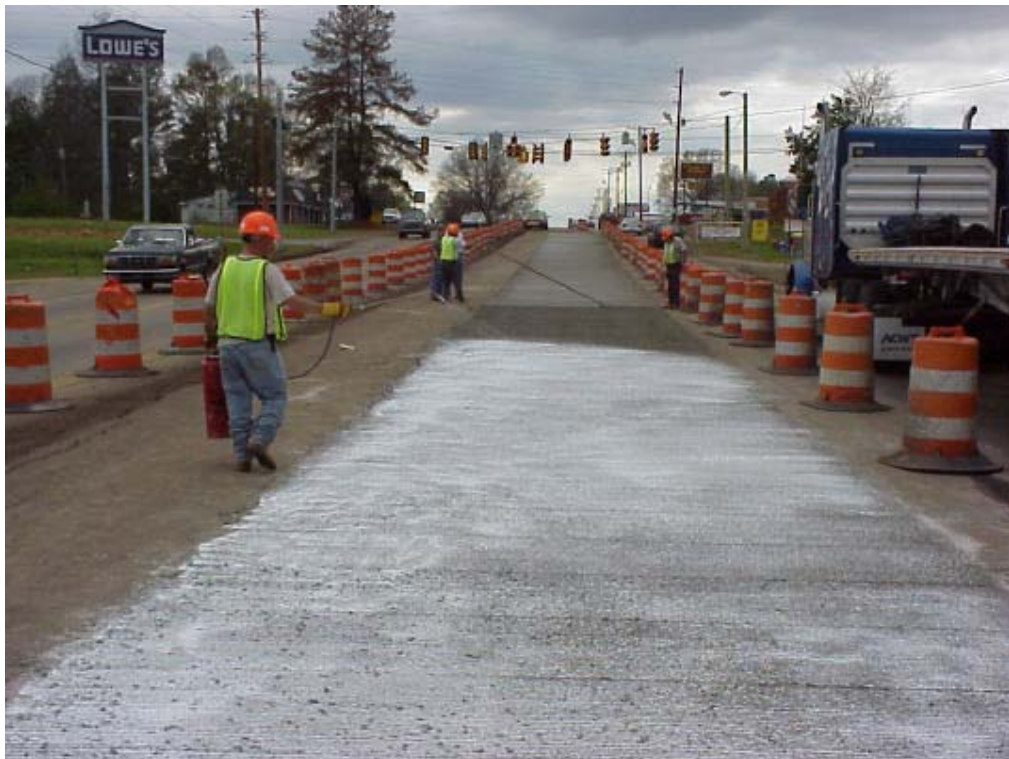
Figure 13 – White pigmented curing compound is applied to fresh concrete
