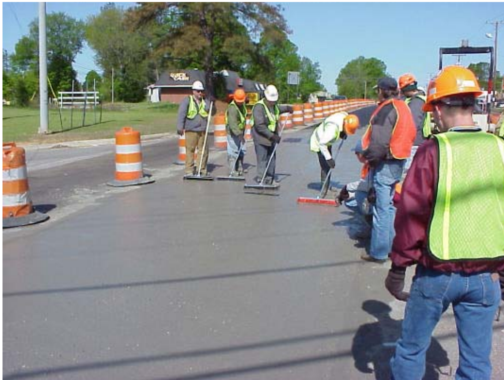
Figure 29 – Excess grout is pulled forward
