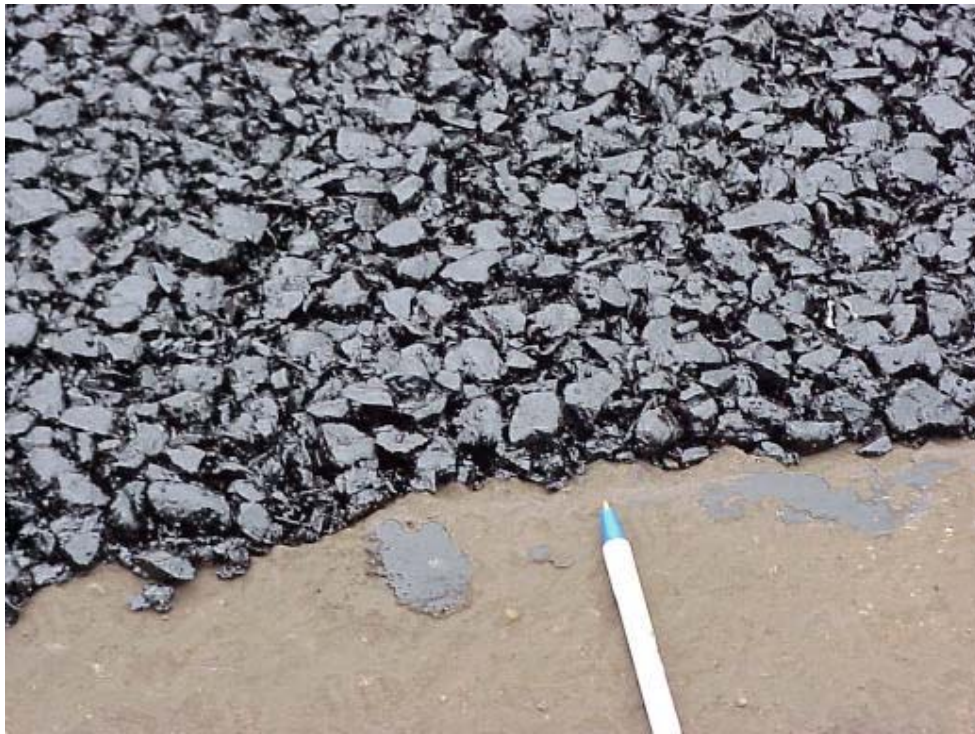
Figure 18 – Close up of the surface of the 2” thick open graded mat
