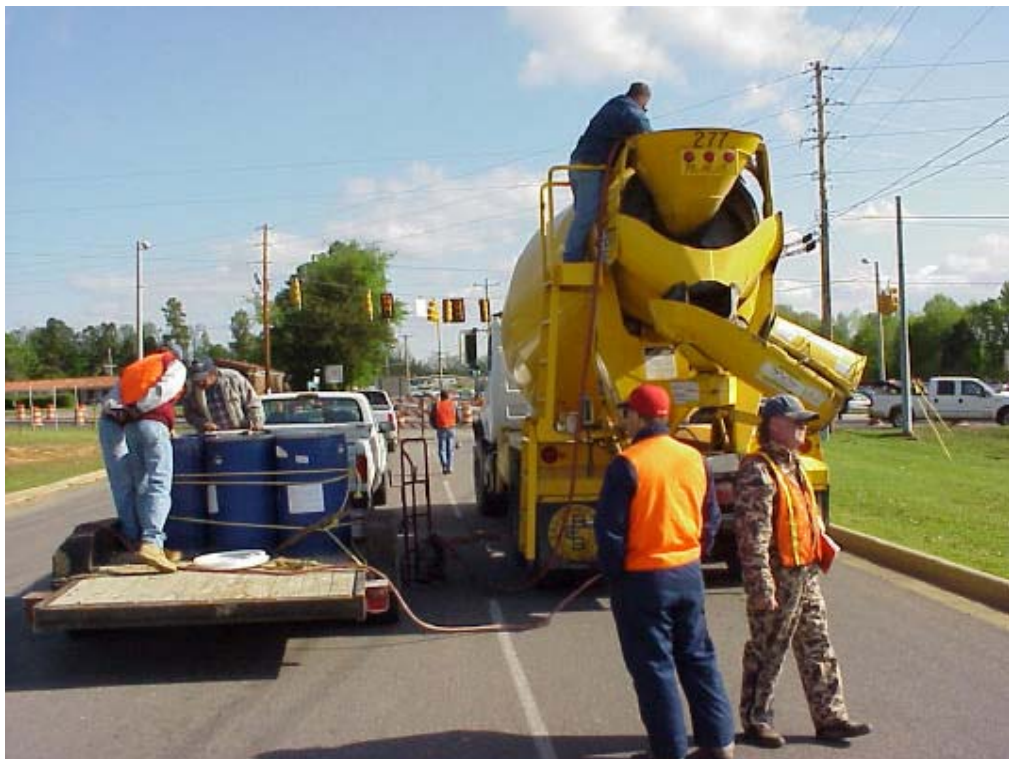
Figure 21 – PL7 latex additive is added to the grout at the site
