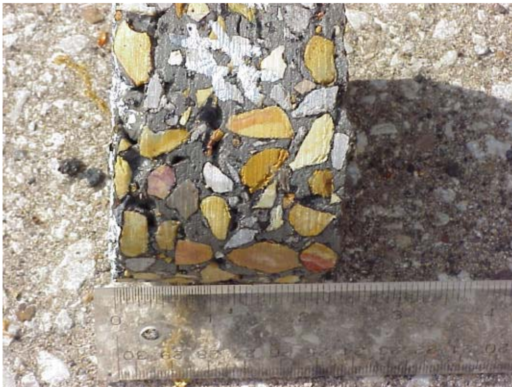
Figure 31 – Cores are taken to insure 95% saturation of grout
