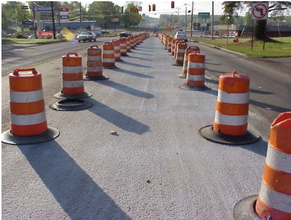
Figure 30 – Finished product the next morning (US 72 & Hinton St. looking east)
