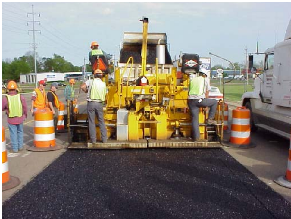
Figure 17 – Paving the PG 67-22 open graded mix for the RMP test section
