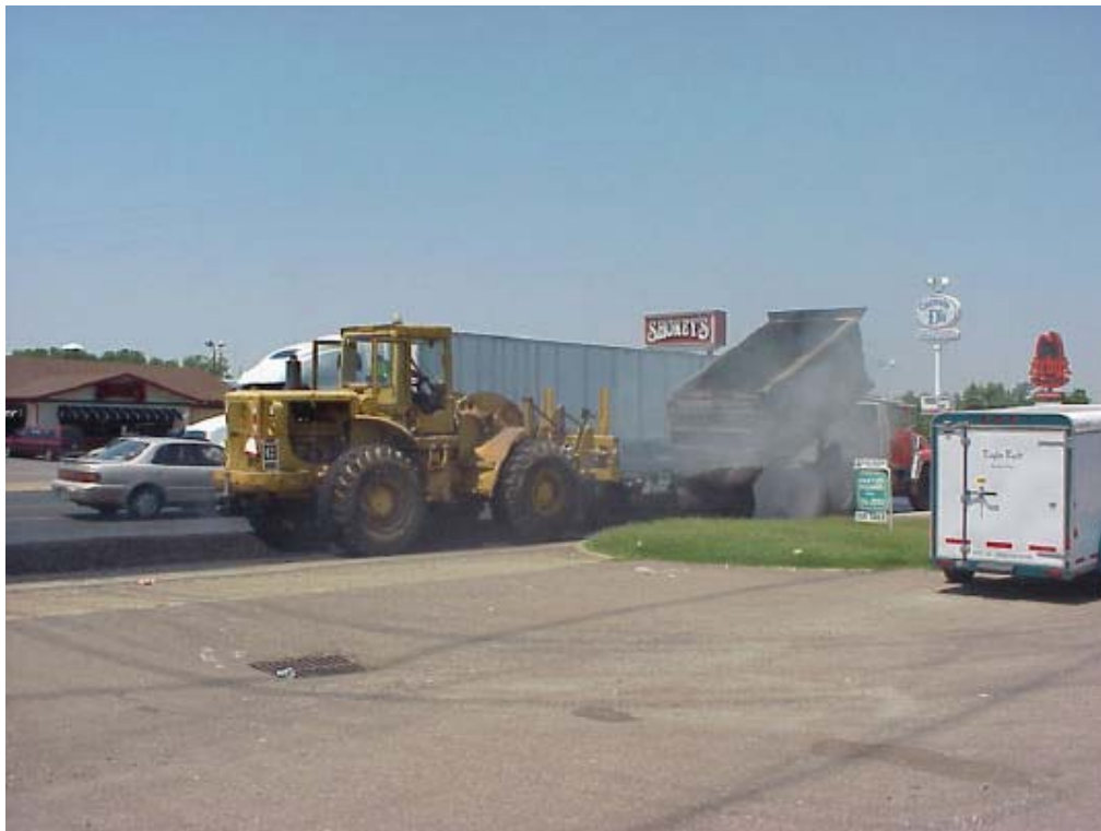
Figure 34 – PG 82-22 dense graded HMA being dumped ahead of Windrow device
