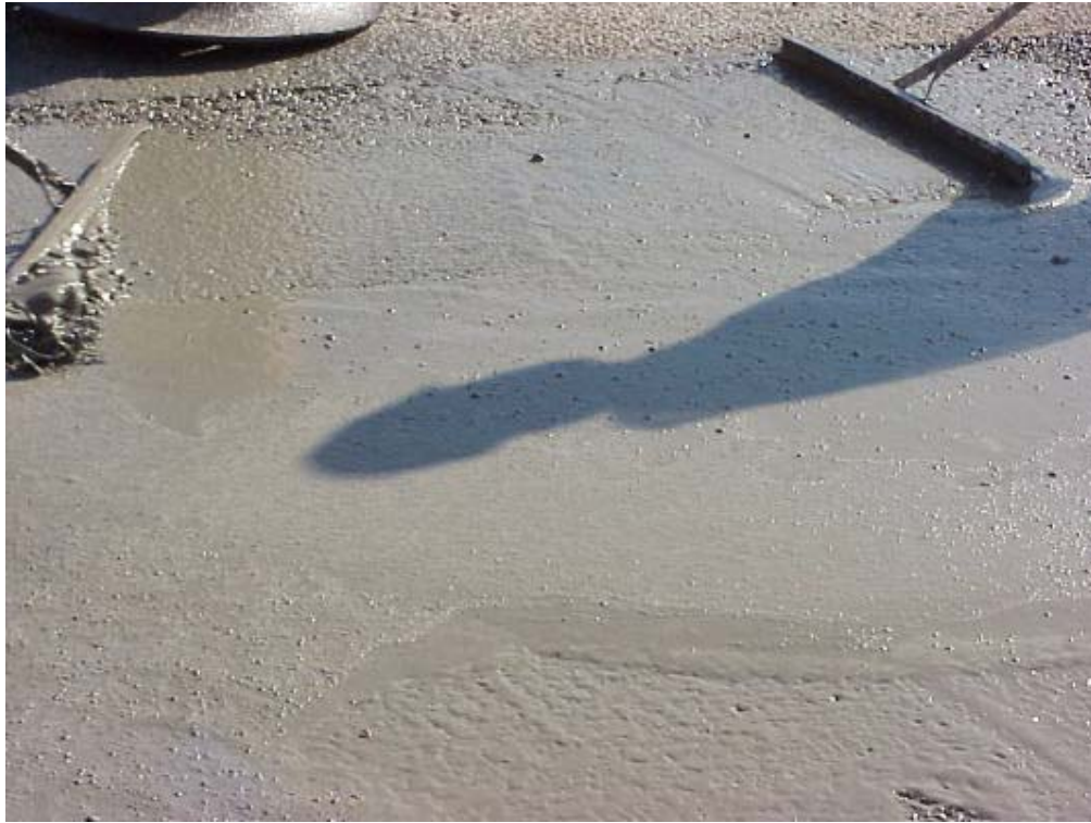
Figure 28 – “Working the grout”
