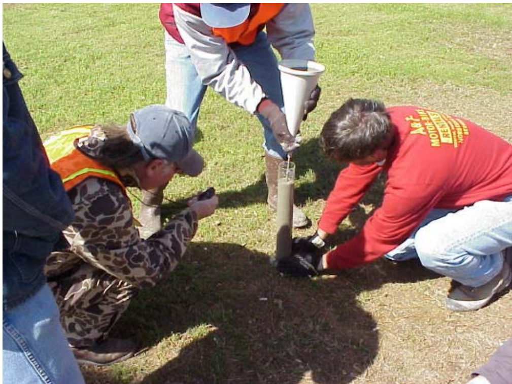
Figure 23 – Flow time of the grout is checked with a Marsh cone
