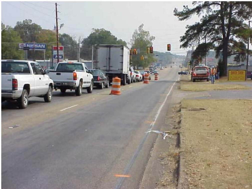
Figure 6 – Intersection of US 72 and Hinton Street (looking east)
