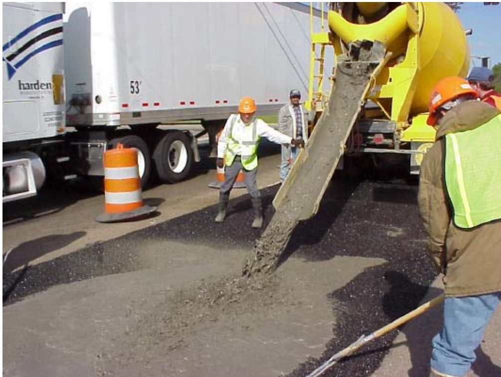
Figure 25 – Grout is poured onto the open graded asphalt mat
