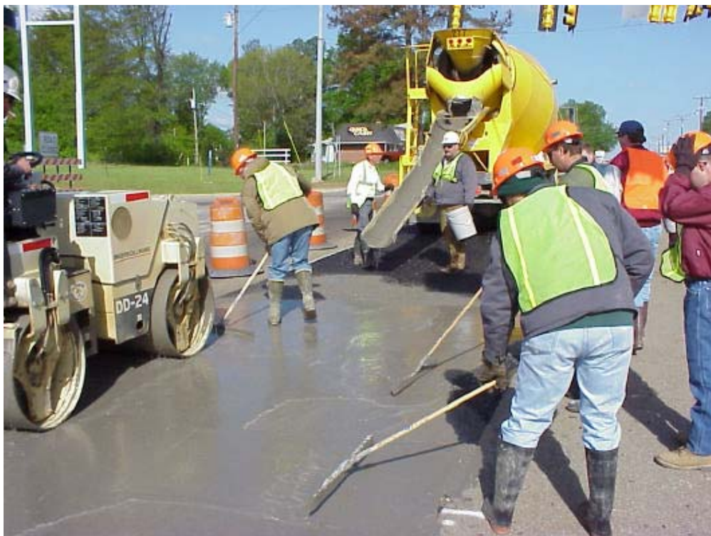
Figure 27 – Excess grout is worked to under grouted areas using squeegees
