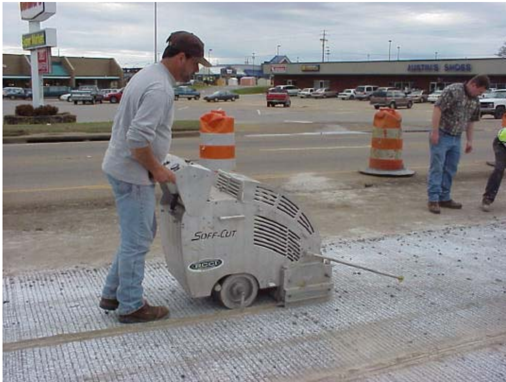
Figure 14 – 3'x3' panels are sawcut into the “green” concrete
