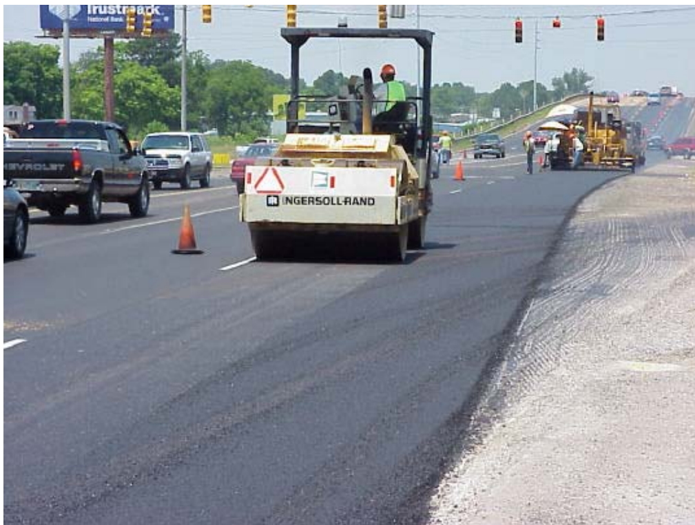
Figure 36 – Breakdown rolling (note scarring from traffic getting on the fresh mat)
