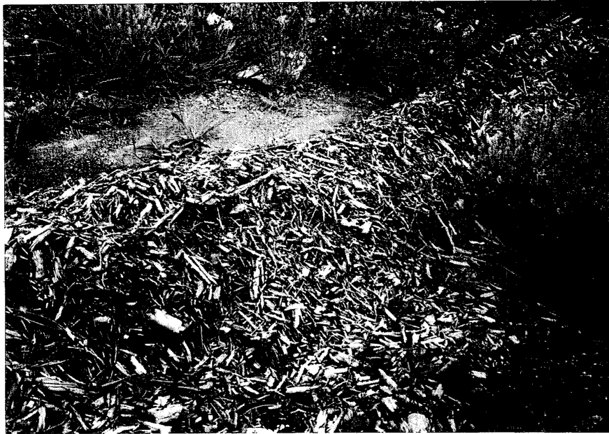
Figure 8.6: Close-up of Filter Berm
