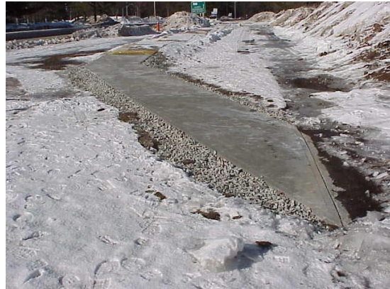
Ramp uncovered on February 26, 2003
