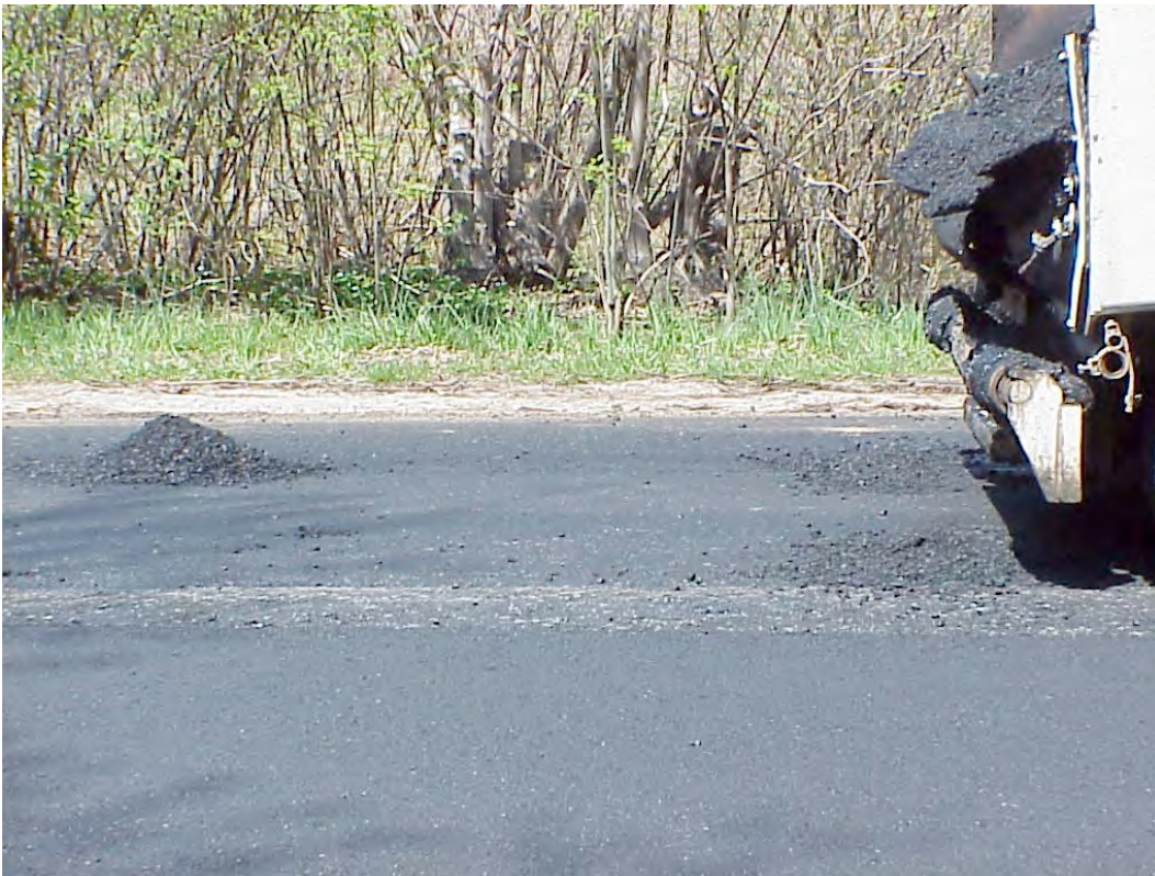
Figure 34. Material Spilled By Truck Pull-Out After Discharge into Paver.
