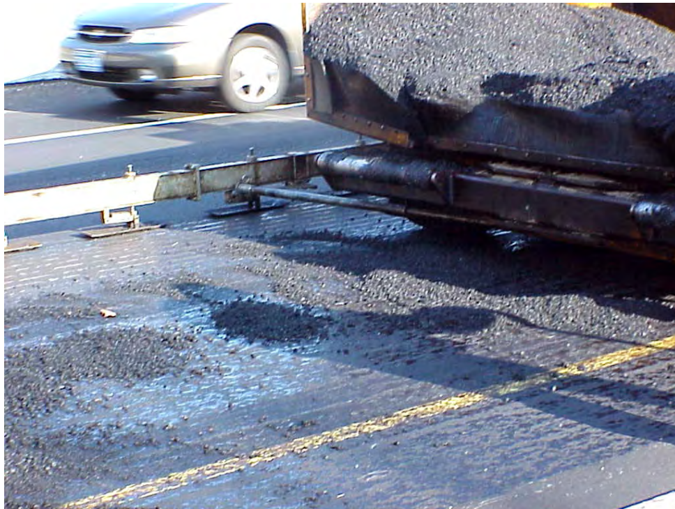
Spillage of Material in Front of Paver and Out of Hopper Bed
