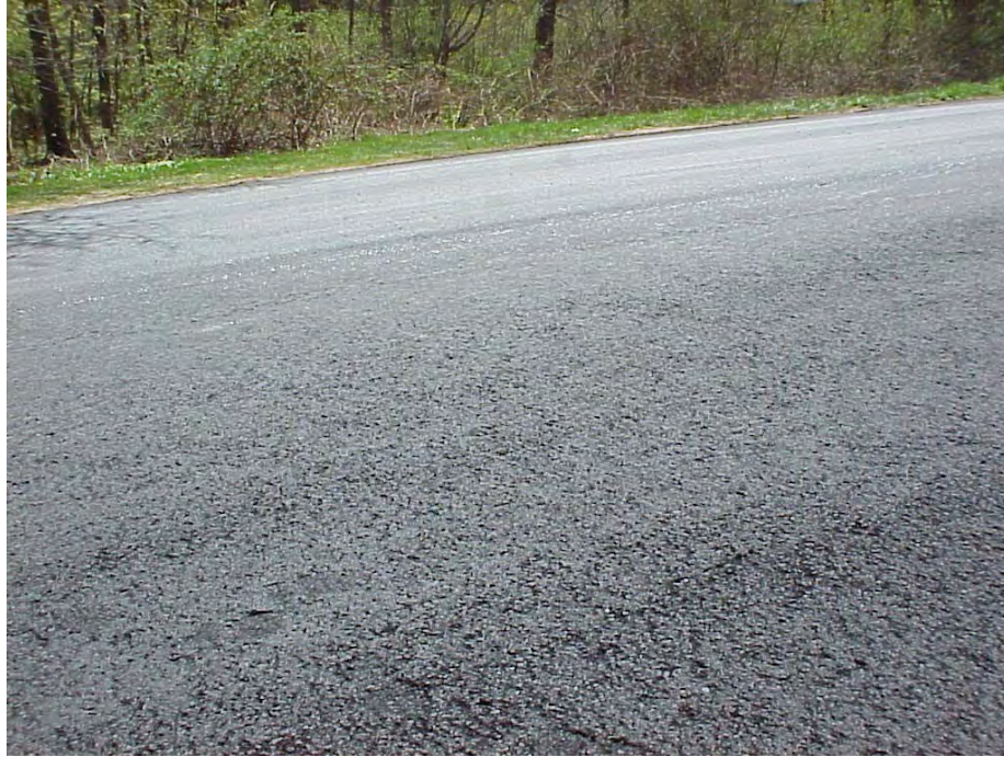
Figure A12. Open-textured Mat Observed Prior to Compaction.
