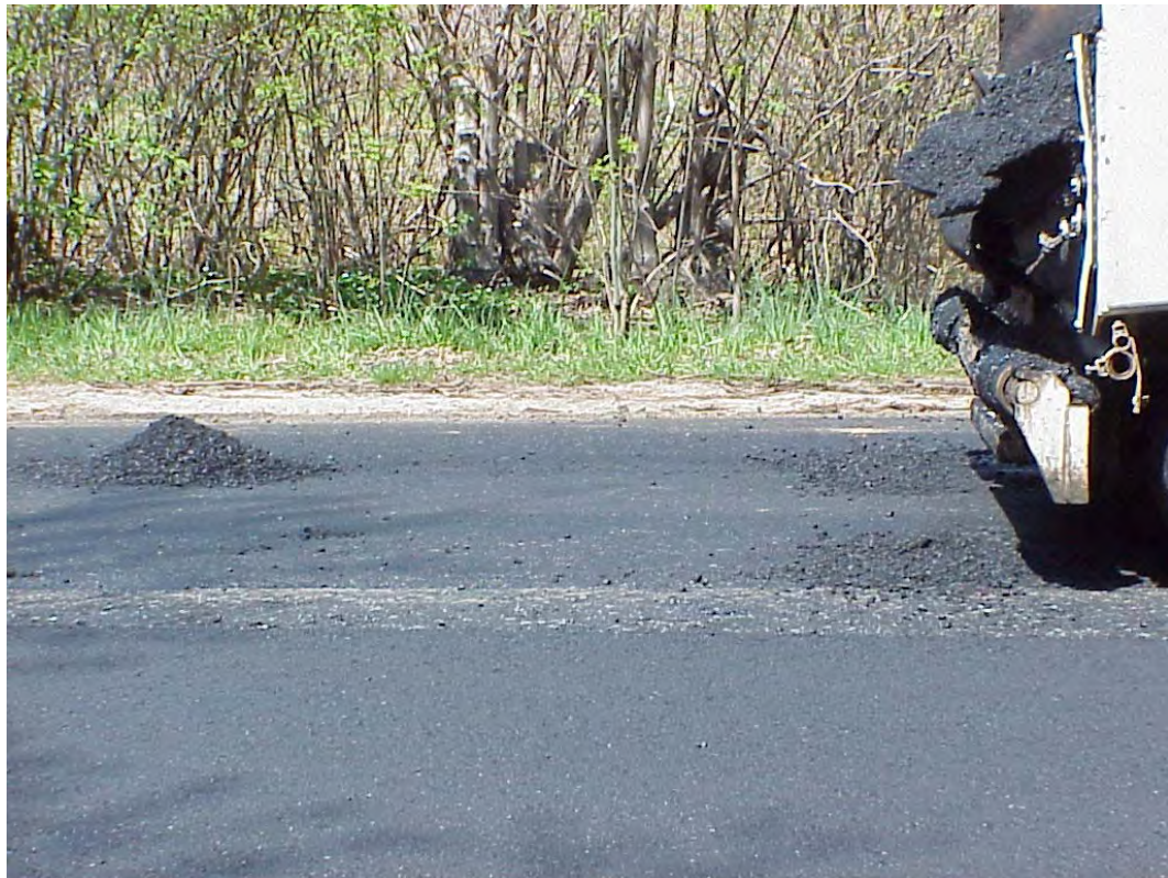
Figure A9. Material Spilled By Truck Pull-Out After Discharge into Paver.
