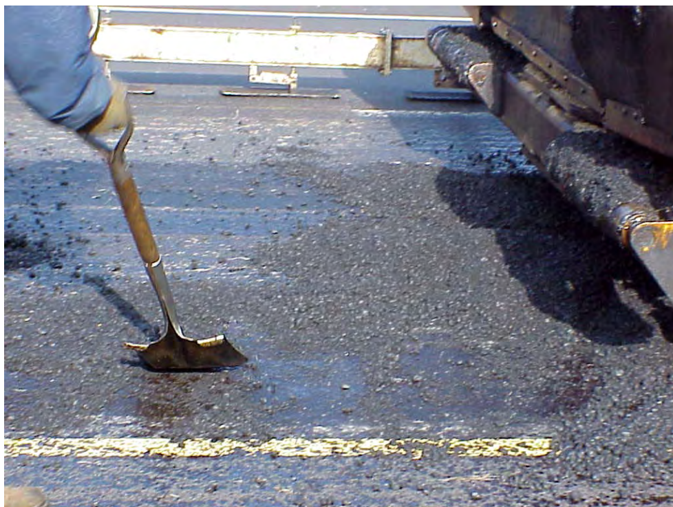
Spillage of Material in Front of Paver and Out of Hopper Bed
