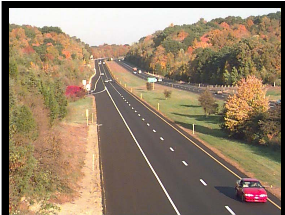
IMAGE #1 - ROUTE 2, BOZRAH/LEBANON TOWN LINE, FACING EAST IN WESTBOUND DIRECTION, SHORTLY AFTER PAVING (SEPTEMBER 1997)
