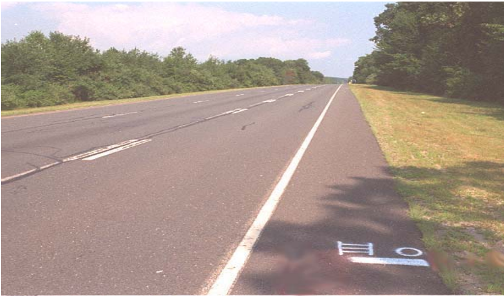
IMAGE #3. ROUTE 2 EASTBOUND PRIOR TO CONSTRUCTION (AUGUST 1996)
