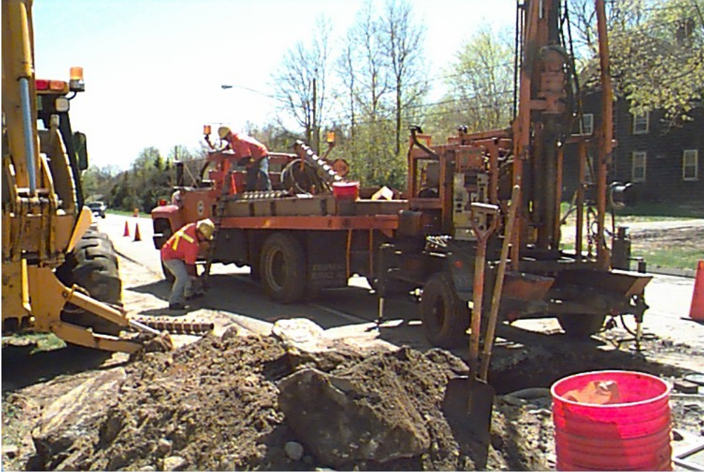
Image 14: Post Seasonal Monitoring Testing, ConnDOT soils sampling (Site 091803)
