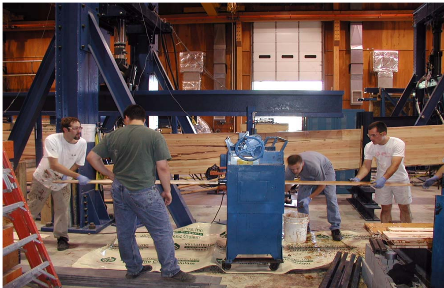
Figure 3.2: Resin Application and Lamination Stacking
