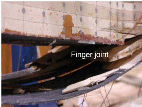
(a) Failure of B1
