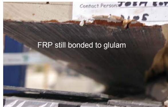
(b) FRP Delamination in B2
