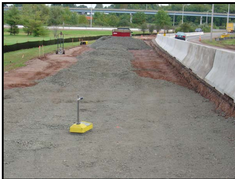
Figure 3.11 I-84 test section, Southington, Connecticut.
