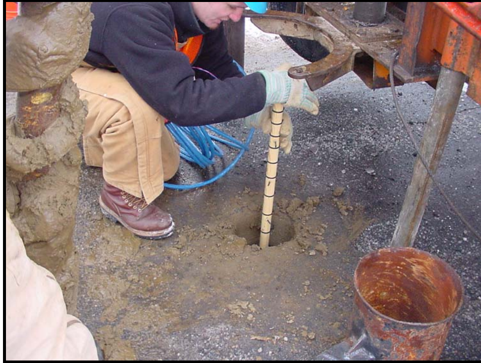
Figure 3.18 Placement of thermocouple string in auger hole.
