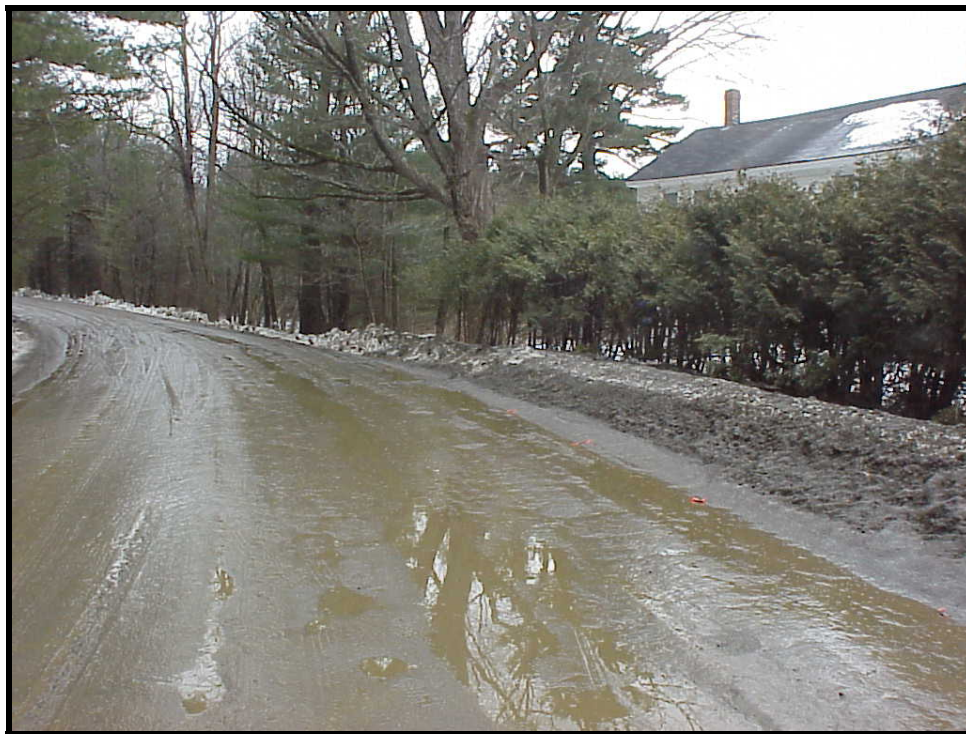
Figure 3.6 Existing conditions at Crosstown Road, Berlin, Vermont in March 2004.
