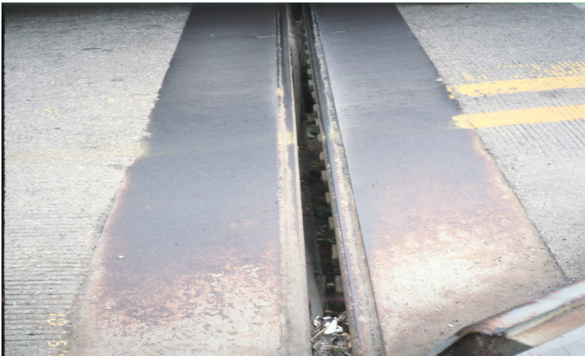
Figure 12. Gland missing.
