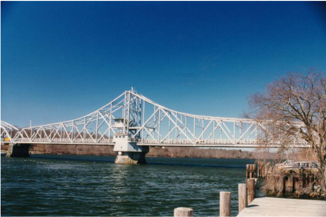
Figure 25 – Old Truss Swing Bridge
