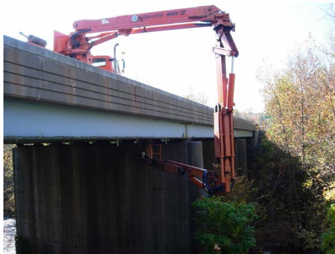
Figure 19 – Installation of Strain Gages on Steel Multi-Girder Bridge
