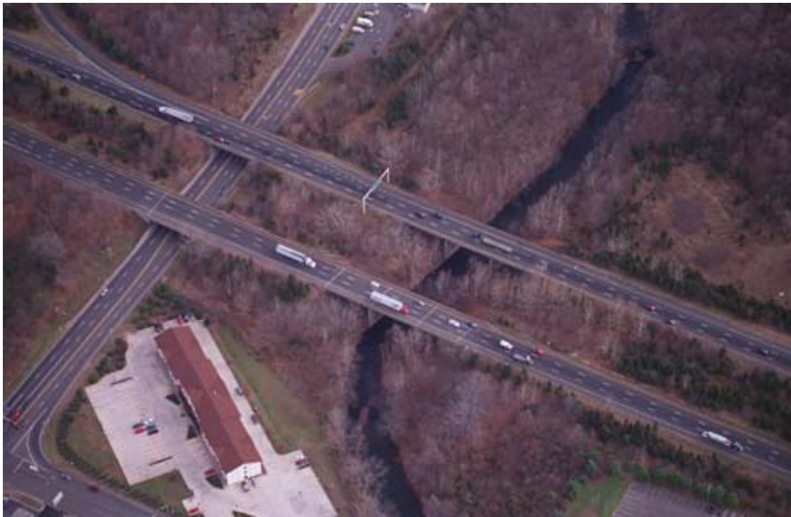
Figure 16 – Aerial View of Steel Multi-Girder Bridge
