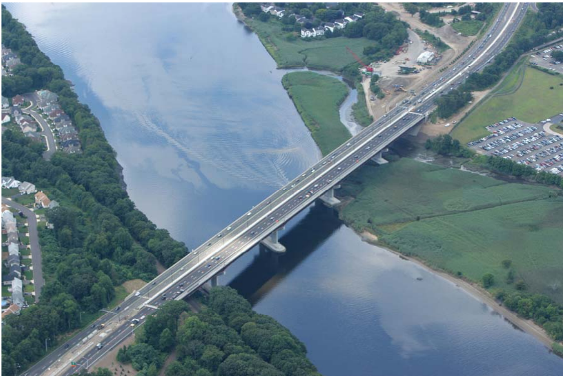
Figure 22 – Multi-Steel-Plate Girder Bridge
