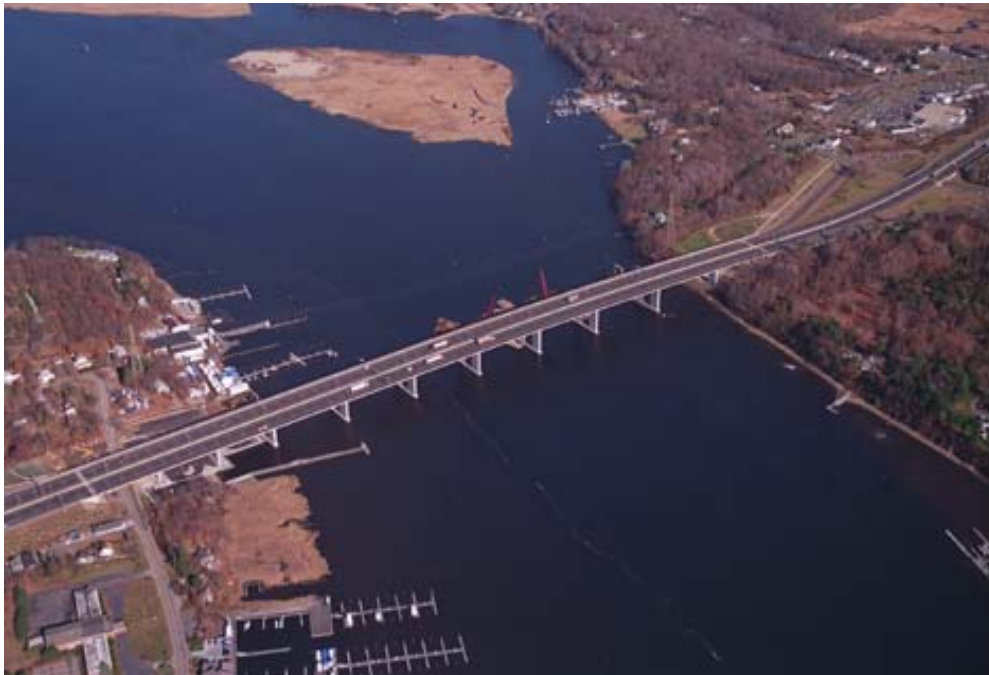
Figure 8 – Aerial View of Post-Tensioned Segmental Box Girder Bridge
