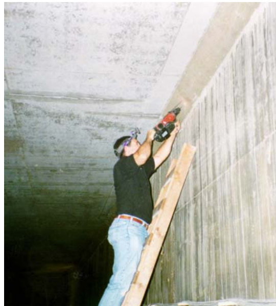
Figure 7 – Installation of Temperature Sensor on Post-Tensioned Box Girder Bridge
