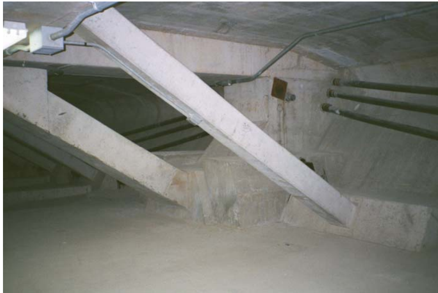
Figure 11 – Interior of Post-Tensioned Segmental Box Girder Bridge
