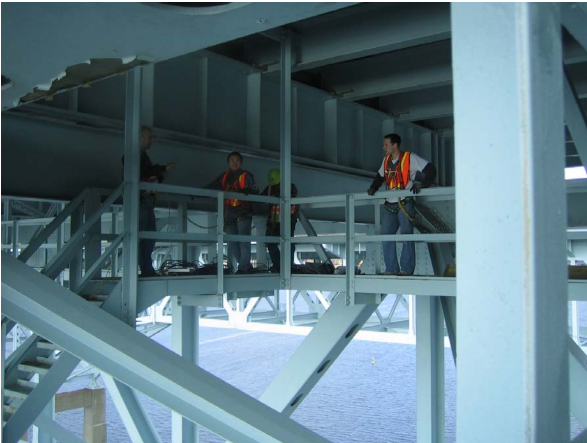
Figure 23 - Large Multi-Span Steel Truss Bridge with Central Hung Trusses
