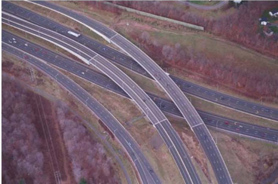
Figure 1 – Aerial View of Post-Tensioned Box Girder Bridge
