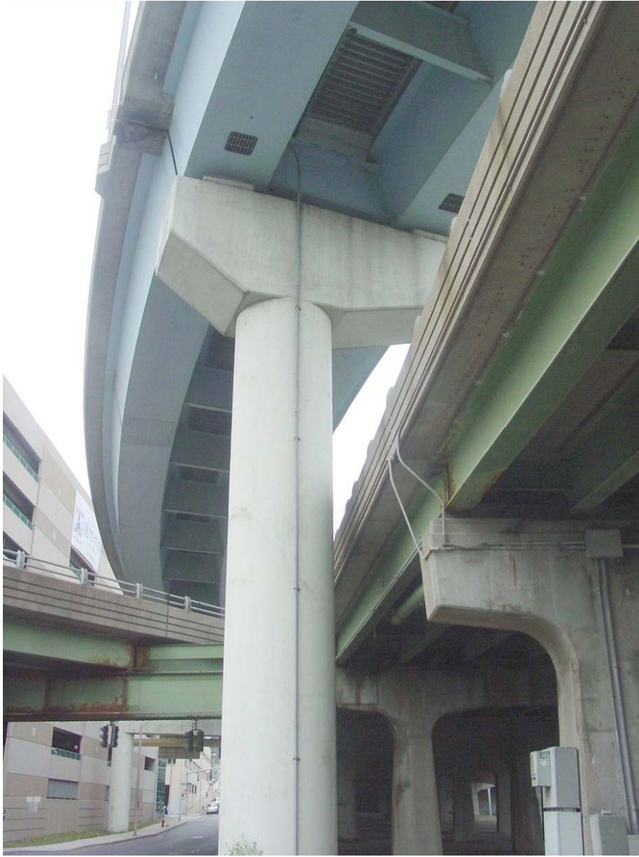
Figure 13 – Support at Pier 3 for Steel Box Girder Bridge
