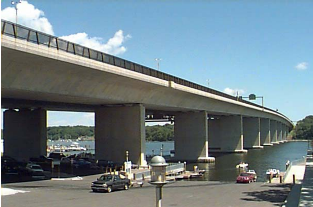
Figure 9 – Elevation of Post-Tensioned Segmental Box Girder Bridge
