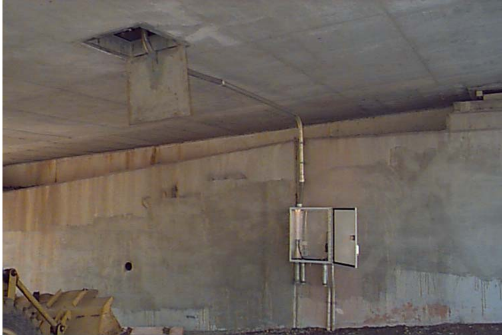
Figure 6 - Enclosure for System Control and Cable Conduit for Post-Tensioned Box Girder Bridge
