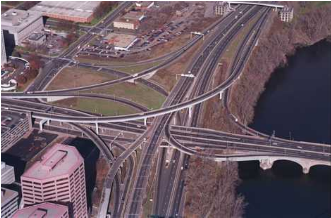
Figure 12 – Aerial View of Steel Box Girder Bridge
