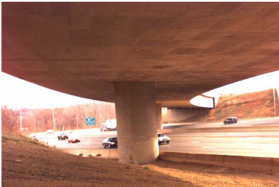
Figure 2 - Underside of Post-Tensioned Box Girder Bridge
