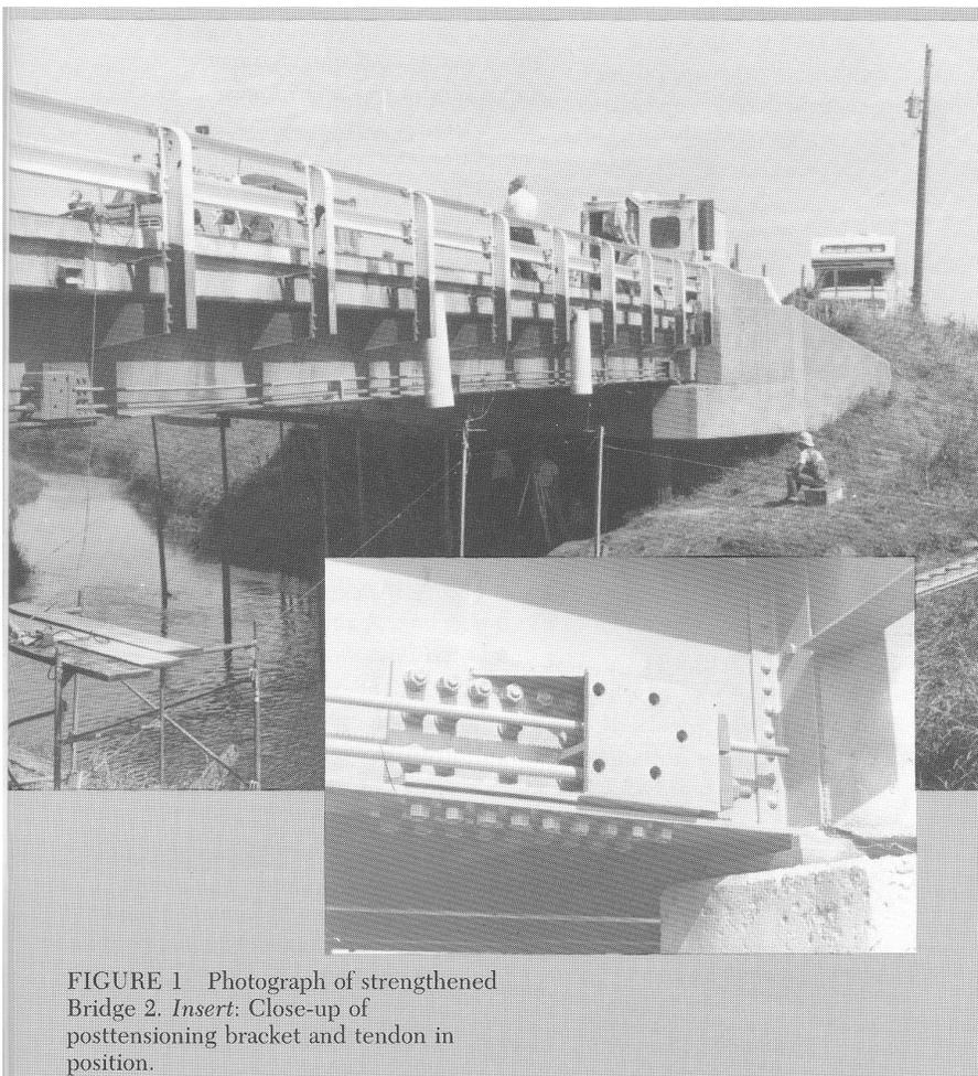
FIGURE 1 Photograph of strengthened Bridge 2. *Insert:* Close-up of posttensioning bracket and tendon in position.
