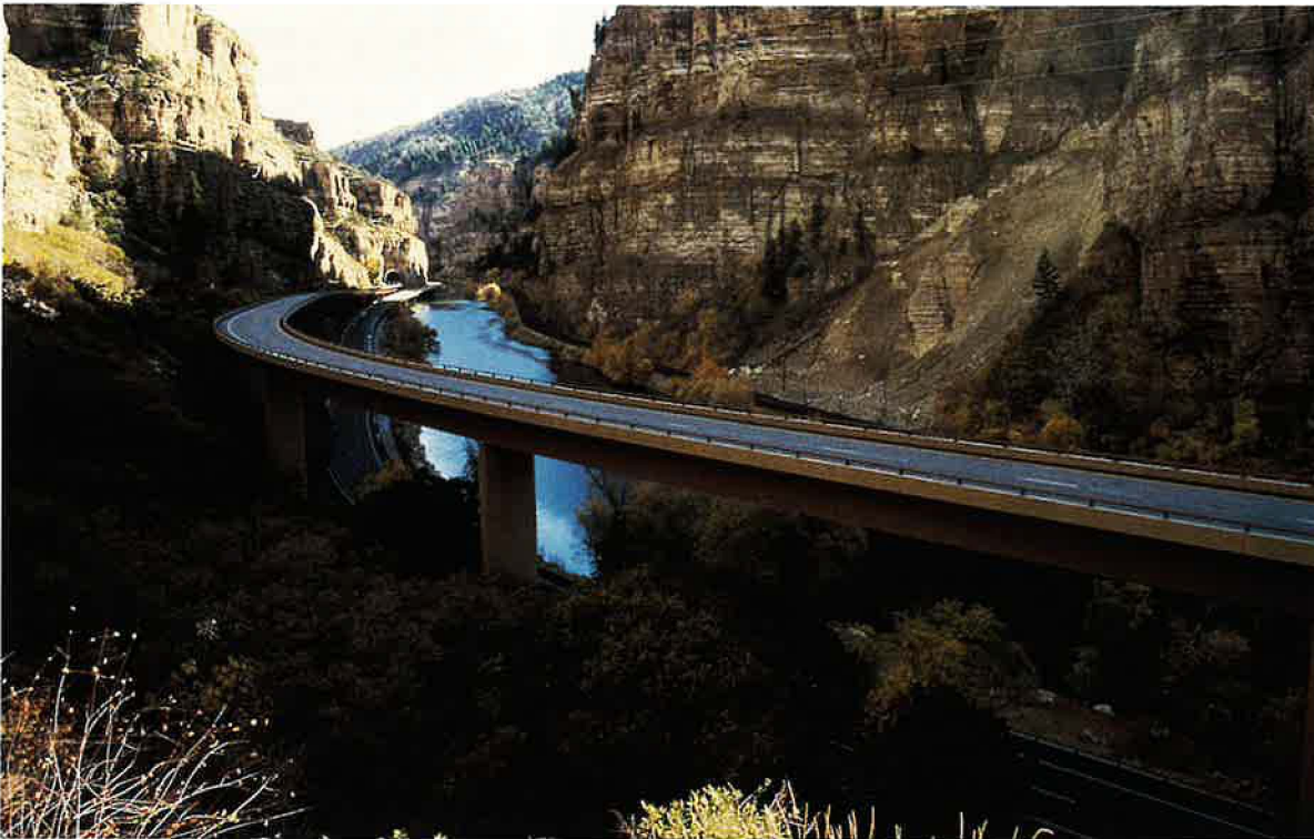
Interstate 70 in scenic Glenwood Canyon, Colorado, was constructed through rugged terrain with minimal environmental damage. The Hanging Lake Viaduct is one of several viaducts constructed in a steep, narrow area with the aid of an overhead gantry that lowered precast concrete segments in place without scarring the landscape.
