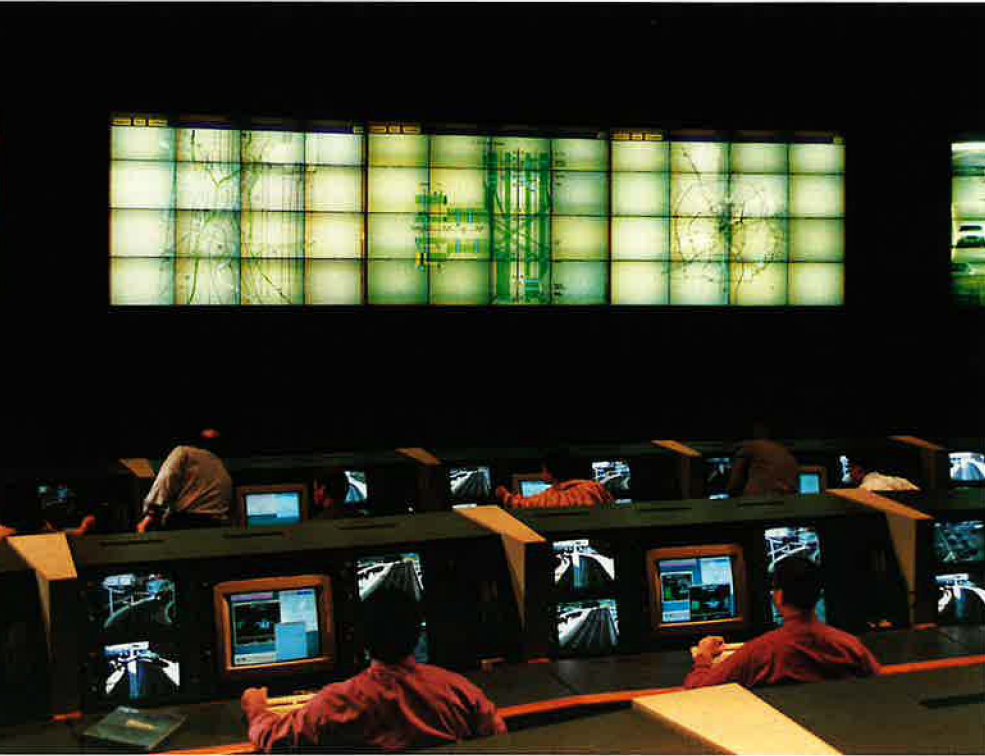
Changeable highway message signs warning of accident or congestion ahead originate in control rooms. Receiving information from a variety of sources, ranging from sophisticated road sensors to calls from drivers, operators at computer terminals alert drivers about traffic and road conditions and suggest alternate routes.
