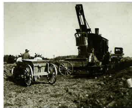
Road building in 1915, using a steam shovel for excavation. After World War I, the nation's energies turned to road building, and the benefits of research soon became apparent to highway engineers.
