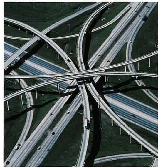
Interchange design has become more complex as the number of vehicles using Interstate highways has increased. Highway engineers began using the trilevel cloverleaf in the 1970s.
