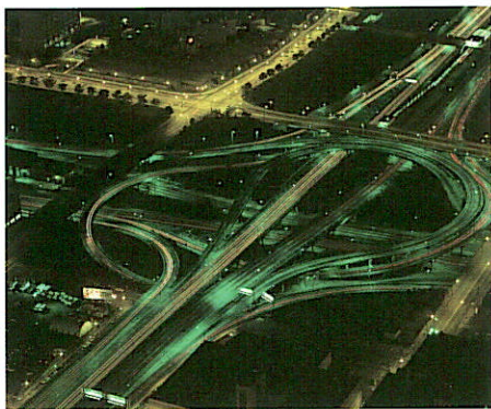
By separating traffic flows, interchanges contribute to safety and increased highway capacity.
