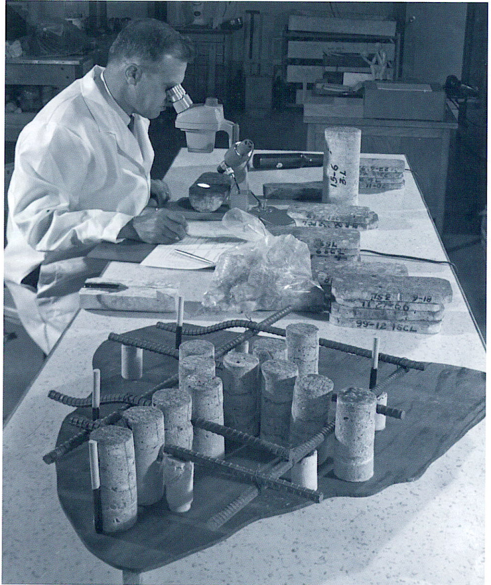
A geologist analyzes concrete pavement cores (circa 1950).
