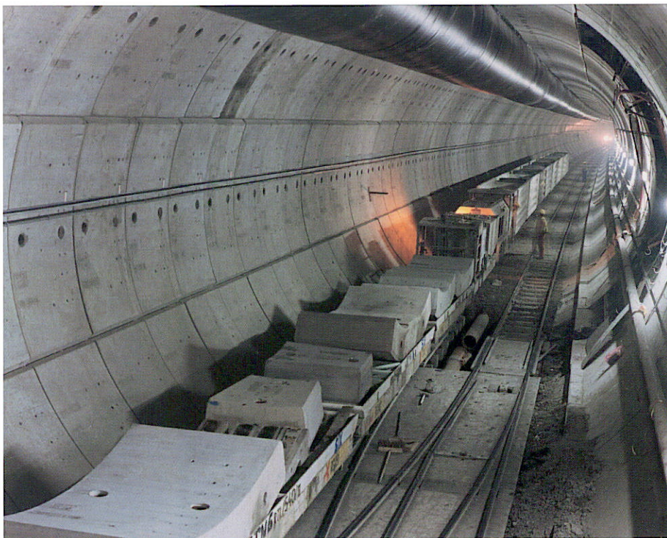
During construction of the Channel Tunnel, connecting England and France, approximately 700,000 segments of reinforced concrete and cast iron were moved in to line the walls, and 7.8 million cubic meters of channel "muck" was moved out. The "chunnel" opened in May 1994.
