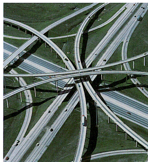
Interchange design has become more complex as the number of vehicles using Interstate highways has increased. Highway engineers began using the trilevel cloverleaf in the 1970s.
