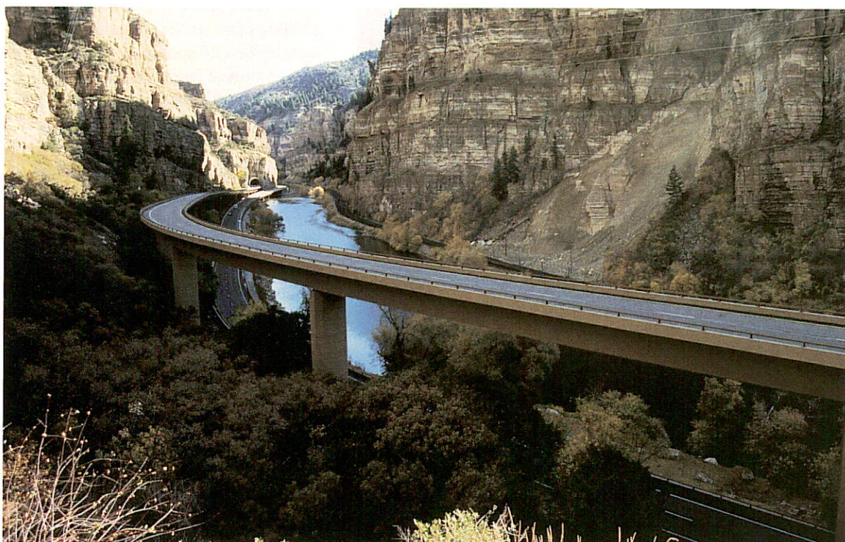
Interstate 70 in scenic Glenwood Canyon, Colorado, was constructed through rugged terrain with minimal environmental damage. The Hanging Lake Viaduct is one of several viaducts constructed in a steep, narrow area with the aid of an overhead gantry that lowered precast concrete segments in place without scarring the landscape.
