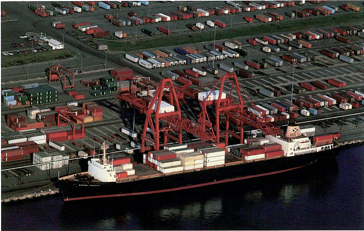
Container ship docked at Norfolk International Terminal. Container ships are integral components of a modern intermodal transport system; containers are efficiently off-loaded to flatcar or truck for delivery. Containerization and sophisticated inland distribution systems have increased speed and efficiency while lowering costs.
