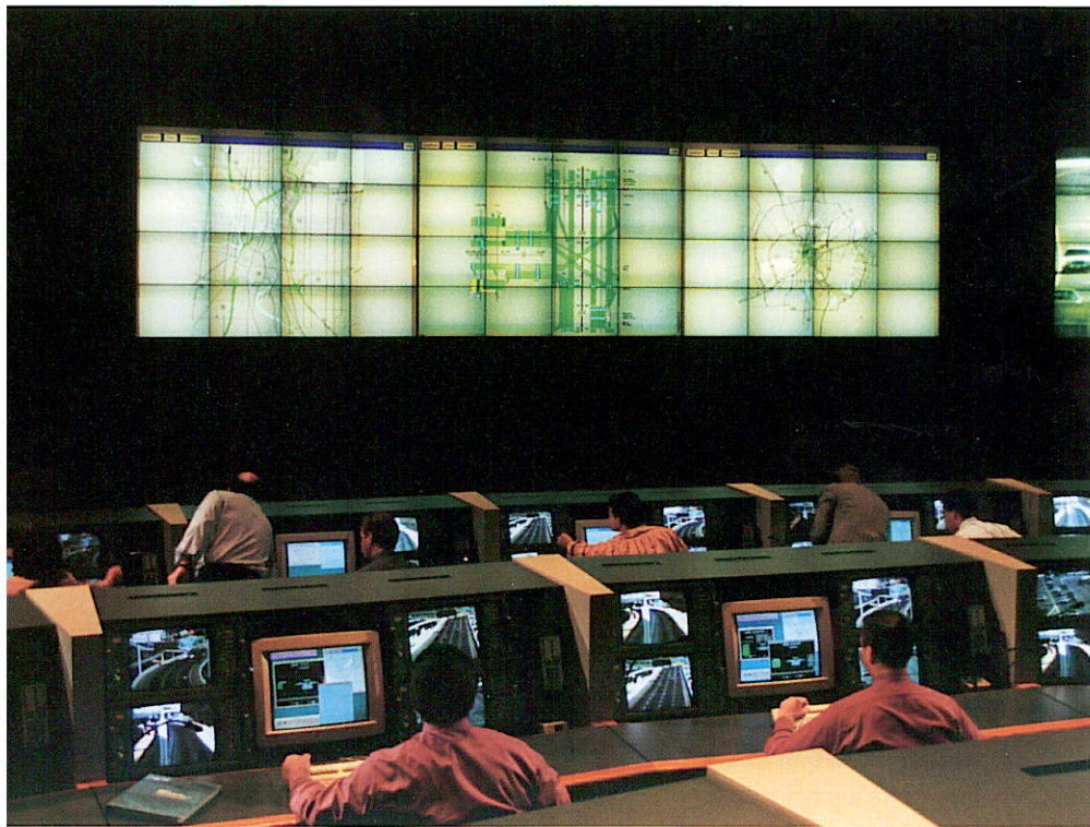
Changeable highway message signs warning of accident or congestion ahead originate in control rooms. Receiving information from a variety of sources, ranging from sophisticated road sensors to calls from drivers, operators at computer terminals alert drivers about traffic and road conditions and suggest alternate routes.
