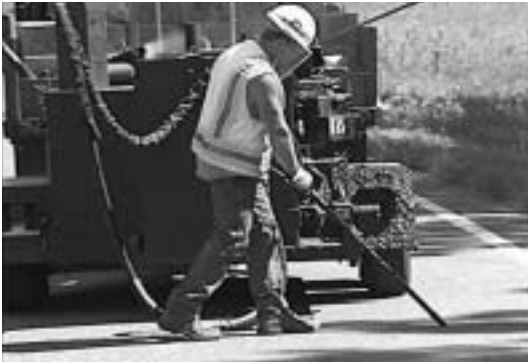
Crack sealing preserves pavement.
