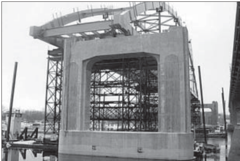
The center arch of bridge, built on the banks of the Mississippi River, is positioned over permanent piers with a mere 7 to 8 inches of clearance; barges then were sunk to drop the arch into place.
