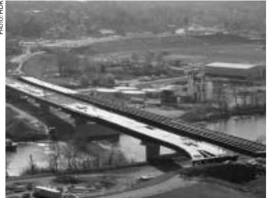
The US-50 bridges in West Virginia were subjected to a value engineering redesign, which saved 1.5 million pounds of steel.
