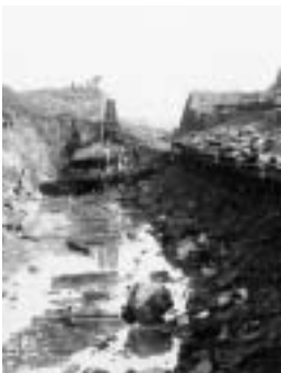
Excavation work during canal construction period.
