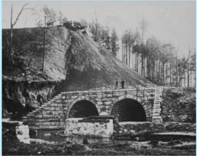
The TRB History Committee seeks to encourage recognition and preservation of historic transportation sites in every state. Above, archival photograph shows construction of the Whiting River Arches, East Canaan, Connecticut, circa 1870. (Photo courtesy of Thomas J. Dodd Research Center, University of Connecticut.)
