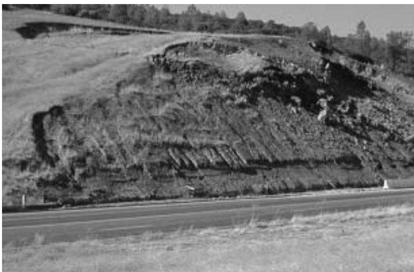
Cut slope failure on Highway 20, Colusa County.
