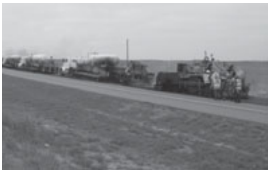
Hot in-place recycling train, with heaters and paver, resurfaces a Kansas road.
