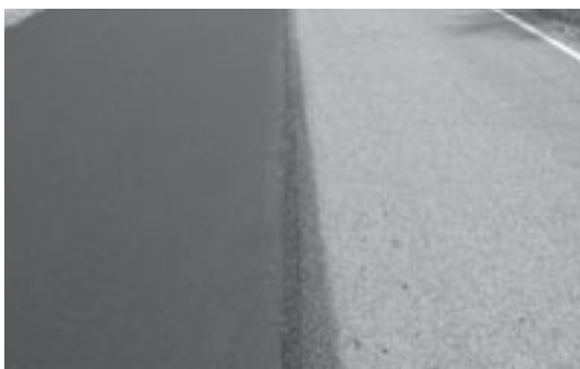
Comparison between a completed lane surface, ready for traffic, after hot in-place recycling (left) with the adjacent lane.
