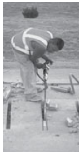
A worker applies a dowel bar retrofit to prevent cracks and faulting in the concrete pavement.
