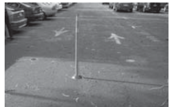
Sensors in the pavement at the parking lot entrance and exit provided a count of space availability.
