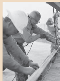
Workers install a guardrail along US-97 during the first stage of the Oregon bridge program.
