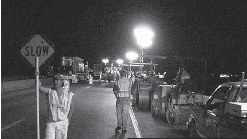
Balloon lighting in use on paving equipment.
