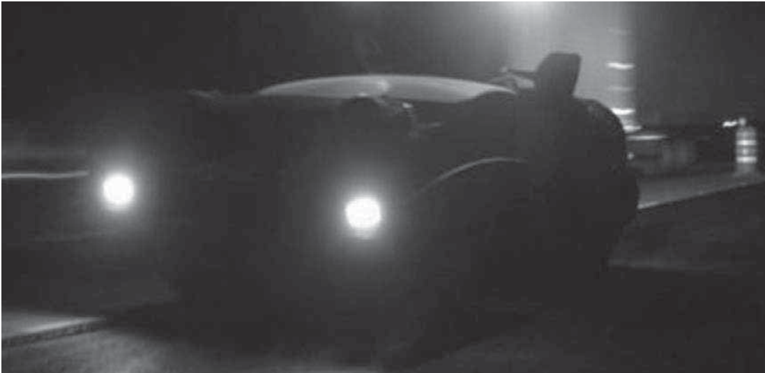
Raised headlights and roller lighting generate a blinding glare for oncoming traffic in the adjacent lane.
