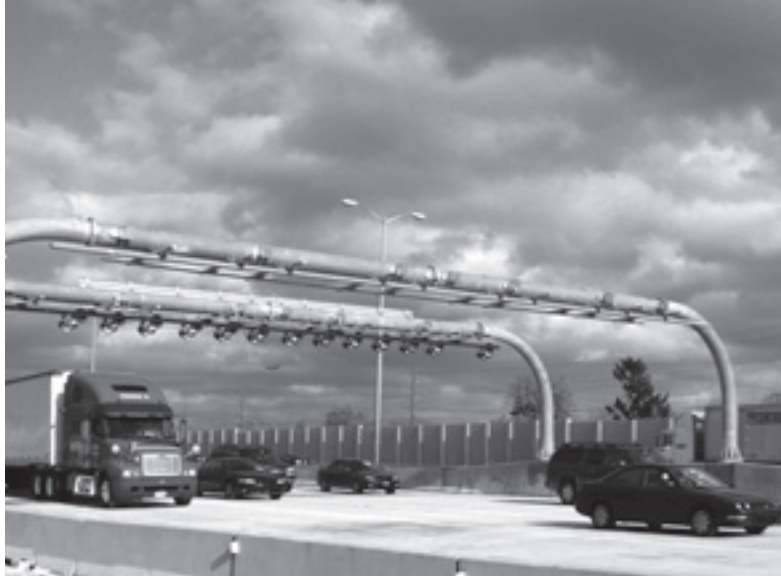
Open road tolling lanes at the Irving Park Road Toll Plaza on the Tri-State Tollway (I-294) in Illinois.
