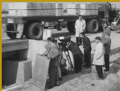
Researchers collect bridge data in the 1955 American Association of State Highway Officials Road Test.
