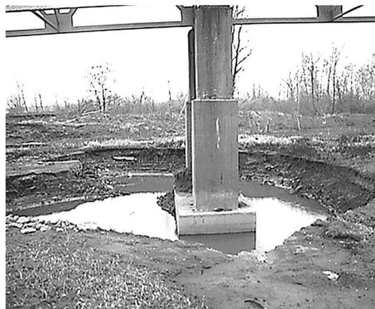
Local sediment scour at a bridge pier in a flood plain after a flow event.
