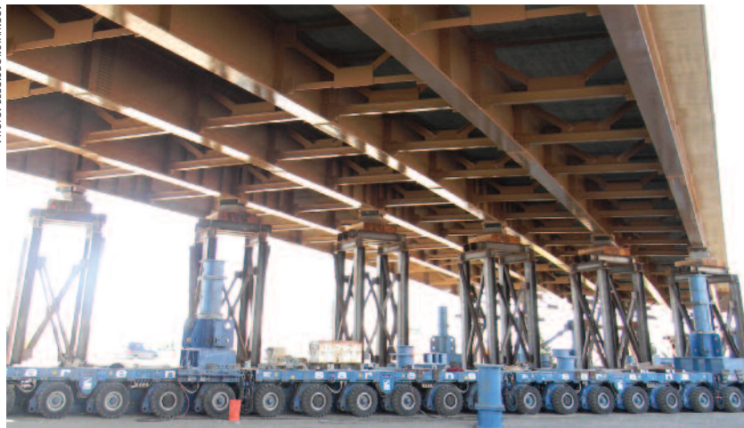
Workers prepare to move the Sam White Bridge near Salt Lake City, using SPMTs.
