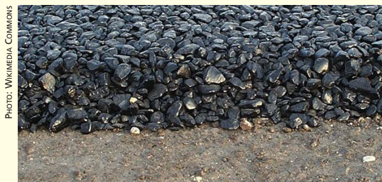
Close-up of an asphaltic concrete layer of a new road under construction.
