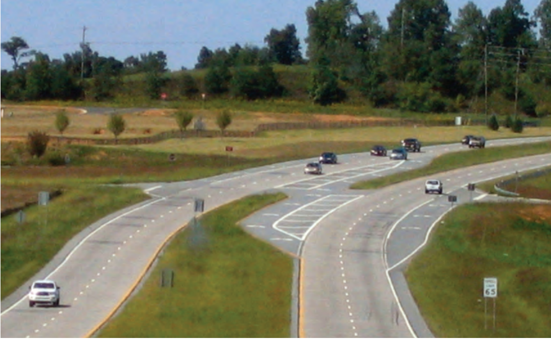
Offset left-turn lanes are the subject of an MRIGlobal study utilizing NDS and roadway data.
