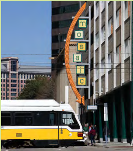
Mosaic Apartments at the Akard Street Dallas Area Rapid Transit station. TCRP projects have explored transit-oriented development and livable communities.
