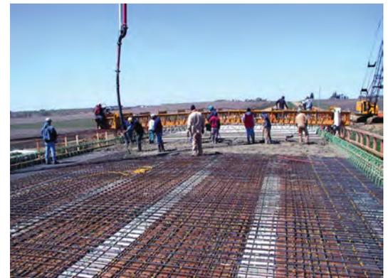
MMFX steel was used in the construction of a bridge deck in Gundy County, Iowa. The developer of the corrosion-resistant and high-strength material began experimenting with dual-phase ferritic martensitic reinforcing steel under an NCHRP IDEA project.
