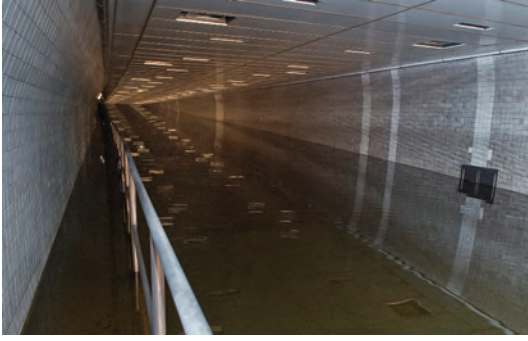
The Hugh L. Carey Tunnel, formerly known as the Brooklyn Battery Tunnel, flooded during Superstorm Sandy. Destruction and severe delays caused many transportation officials to reexamine emergency procedures.
