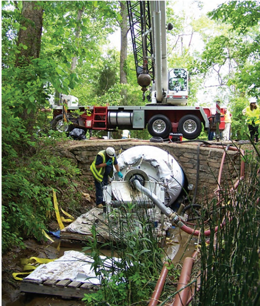
Conventional CIPP steaming process.
