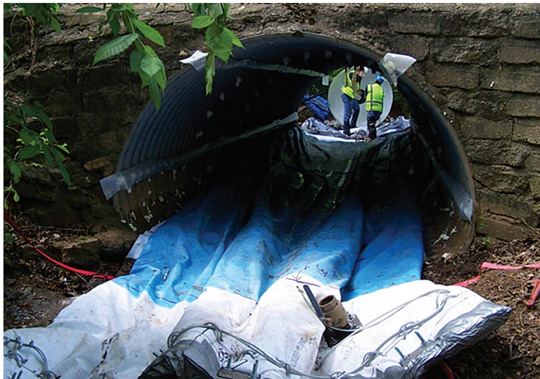
Conventional CIPP liner inserted into host pipe.
