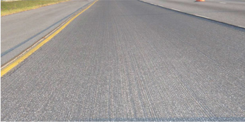
Variable-depth micromilled surface.
