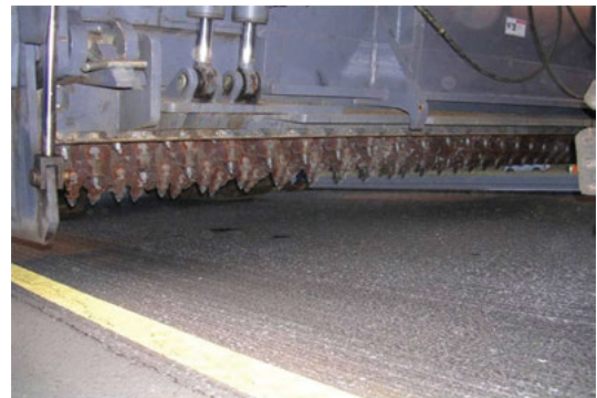
Micromilling operation.
