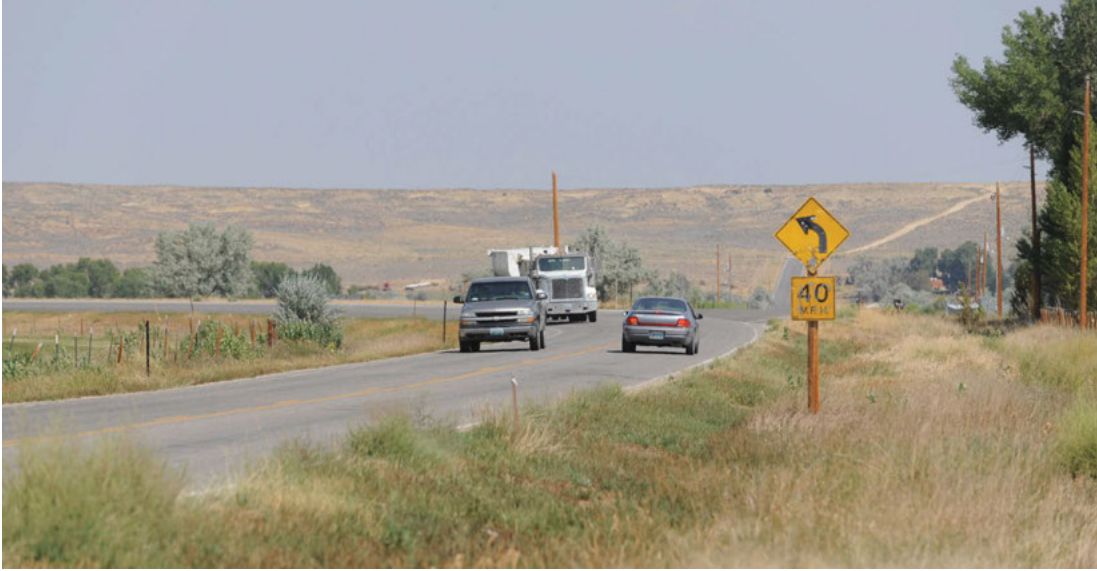
Seventeen Mile Road before construction of safety improvements.
