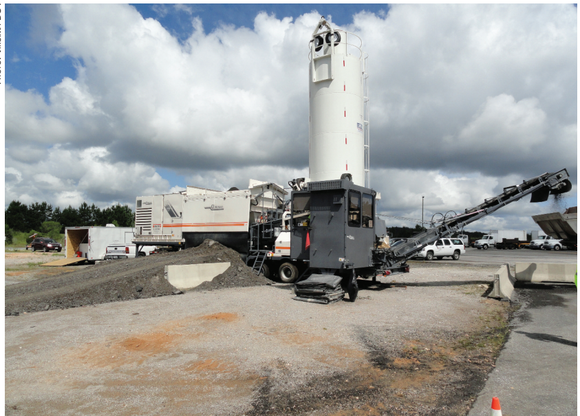
Cold central-plant recycling.
