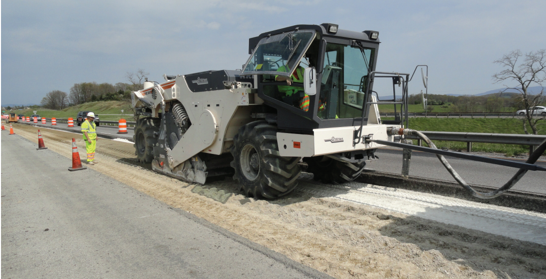
Full-depth reclamation on Interstate 81.
