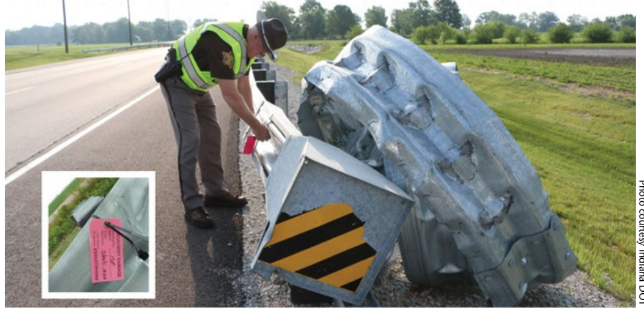
Law enforcement official applying damage tag to infrastructure damaged by motor vehicle crash.
