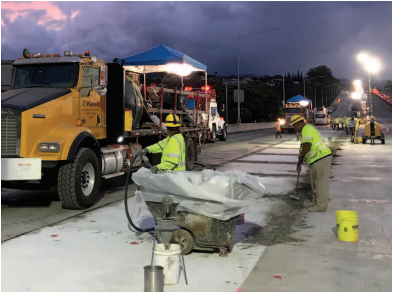
FIGURE 10 Grouting panels after installation. (Source: The Fort Miller Company.)
