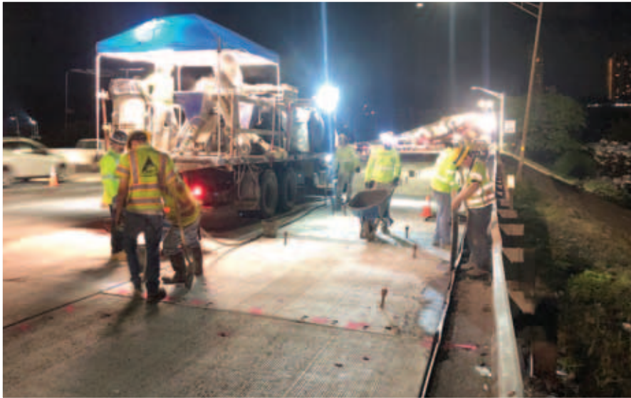
FIGURE 7 Panel elevation adjustment using embedded jacks. (Source: Hawai'i DOT.)
