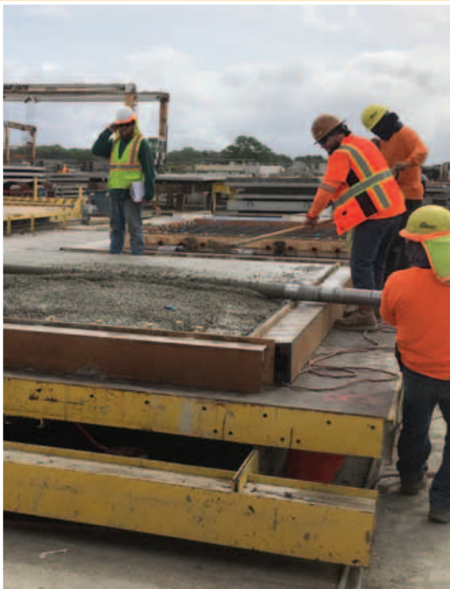
FIGURE 3 Precast panel fabrication for H-1 project. (Source: Hawai'i DOT.)
