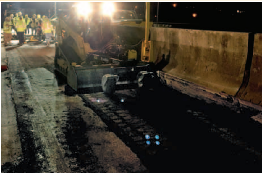
FIGURE 8 Laser screed trimming CTB. (Source: The Fort Miller Company.)
