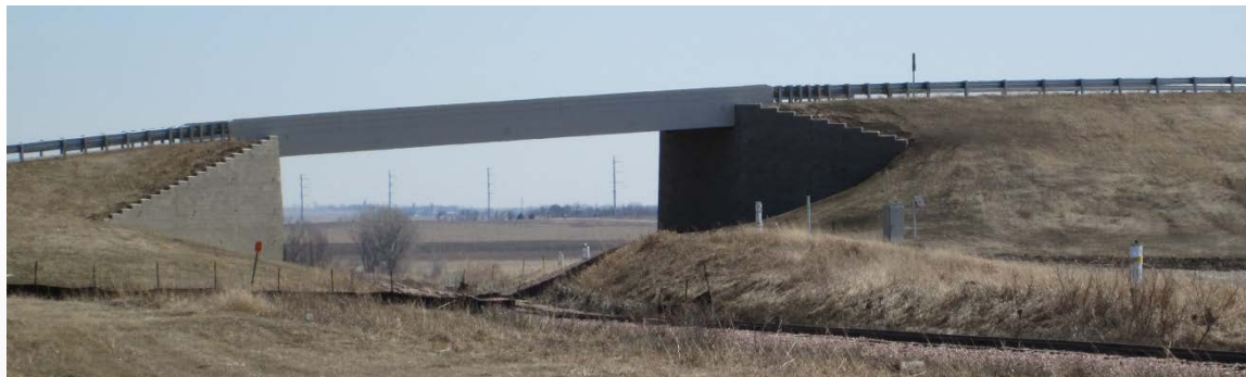
CR 55 over Minnesota Southern RR, MN (2013)
