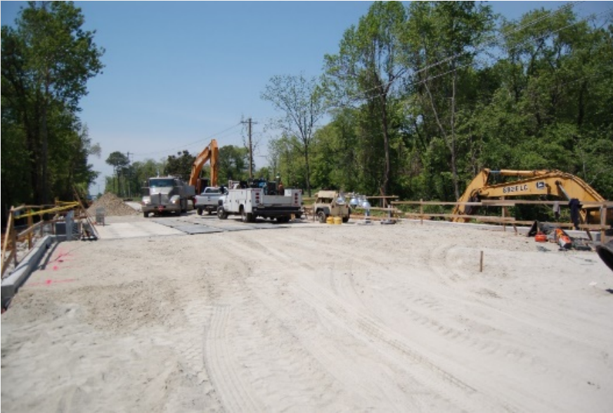
Construction of transition zone
