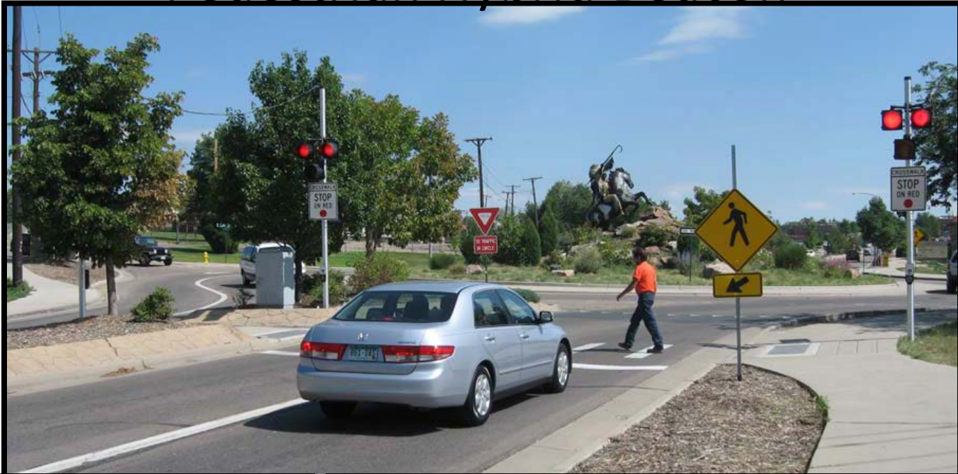
Figure 4F-3. Sequence for a Pedestrian Hybrid Signal
