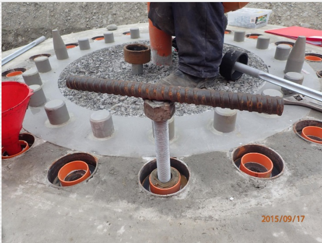
Installing Dissipater Connections
