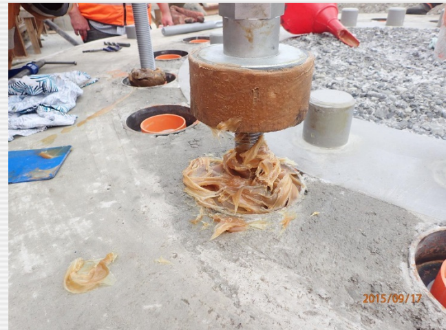
Installing Dissipater Connections
