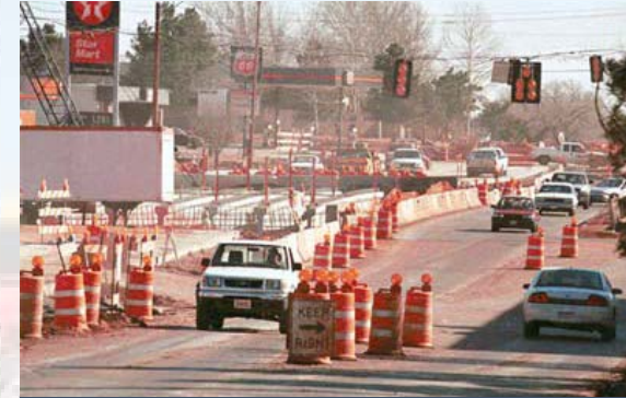
Highway Safety and Reliability
