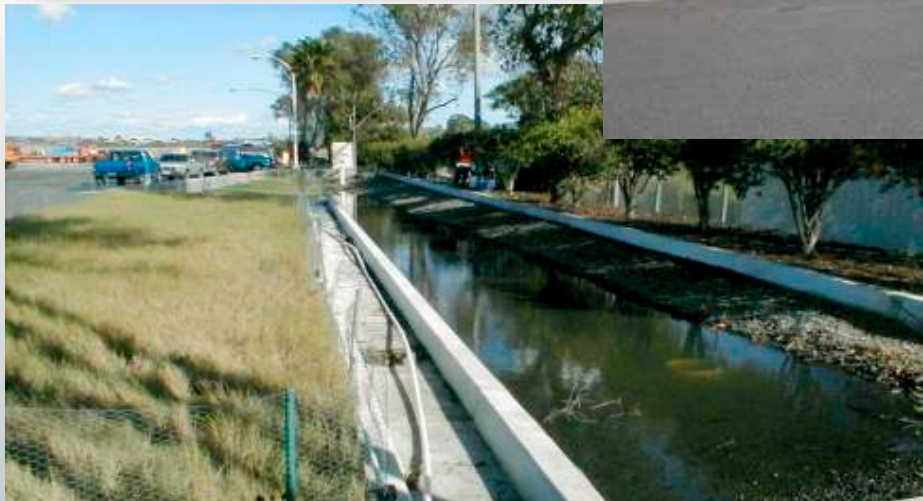
Biofilter Strip/Infiltration Trench
