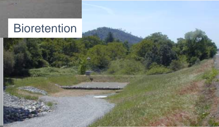
Media Filter – Earthen
