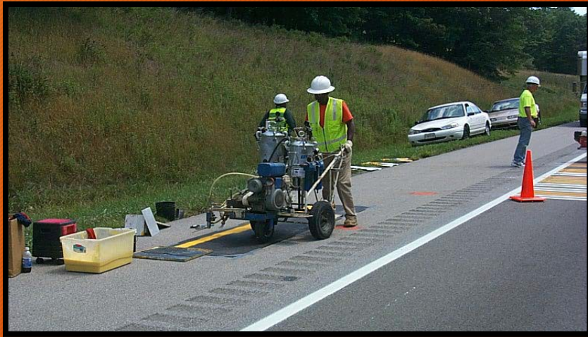
Site Preparation & Equipment Calibrations
