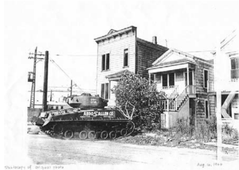
Demolition of West Oakland for Bay Area Rapid Transit
