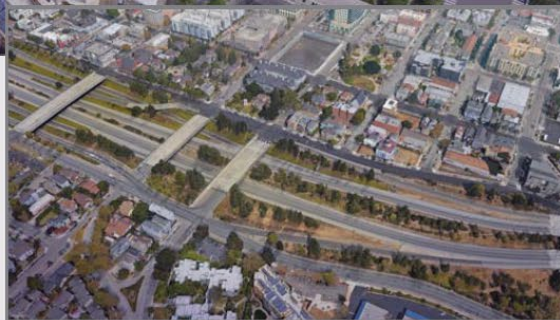
Figure VG-9: Existing I-980 Boulevard
