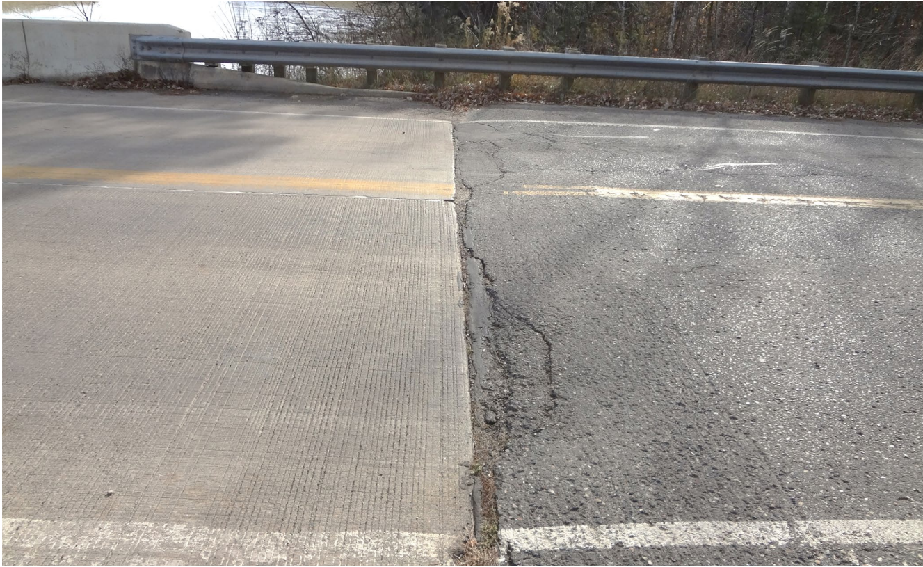
275' Long Bridge , 500 ADT, 20 Years Old
