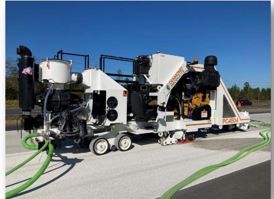
Longitudinal diamond grinding at the US-301 Concrete Test Road
