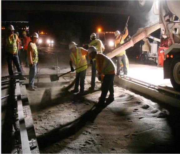
Placement of Bedding Material
