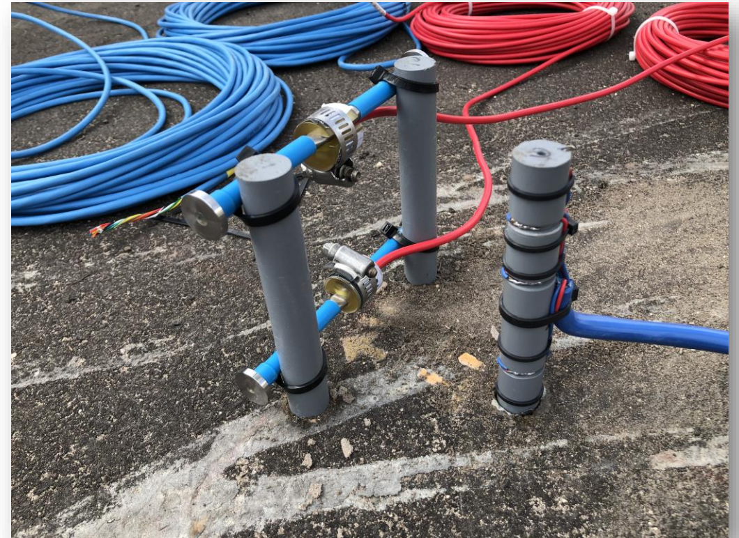
Vibrating wire strain gauges & thermocouple tree
