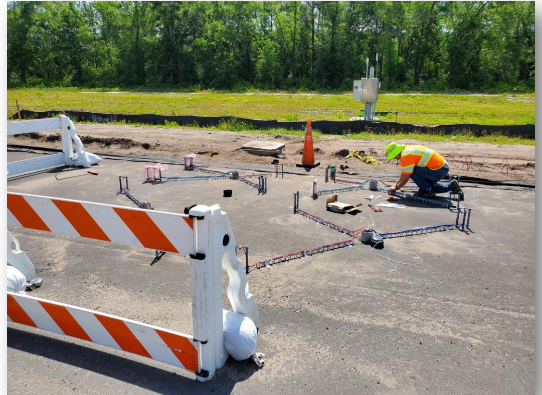
Installing strain gauges & thermocouple trees on US-301
