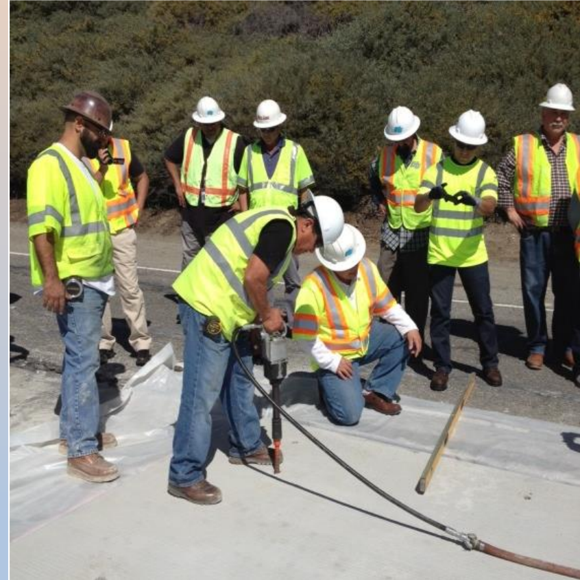
Leveling Screw Grade Control
