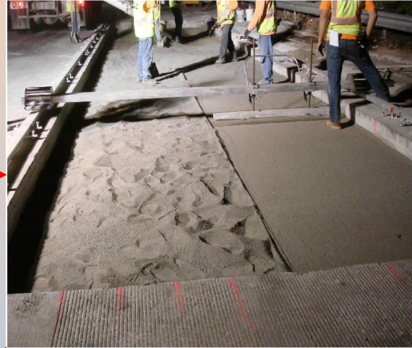
First Grading Pass
