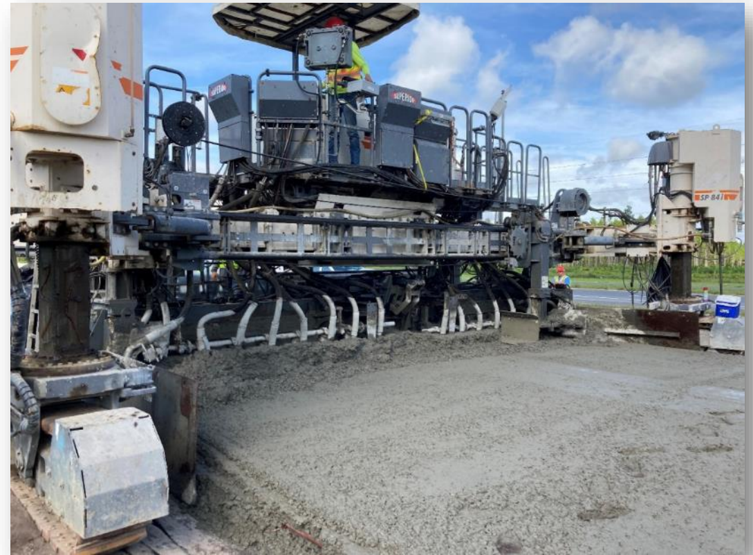
Raise travel lane set of vibrators when near sensors but keep them on
